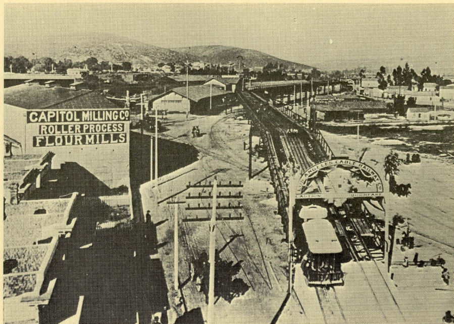
Los Angeles Cable Railway near old River Station of Southern Pacific
