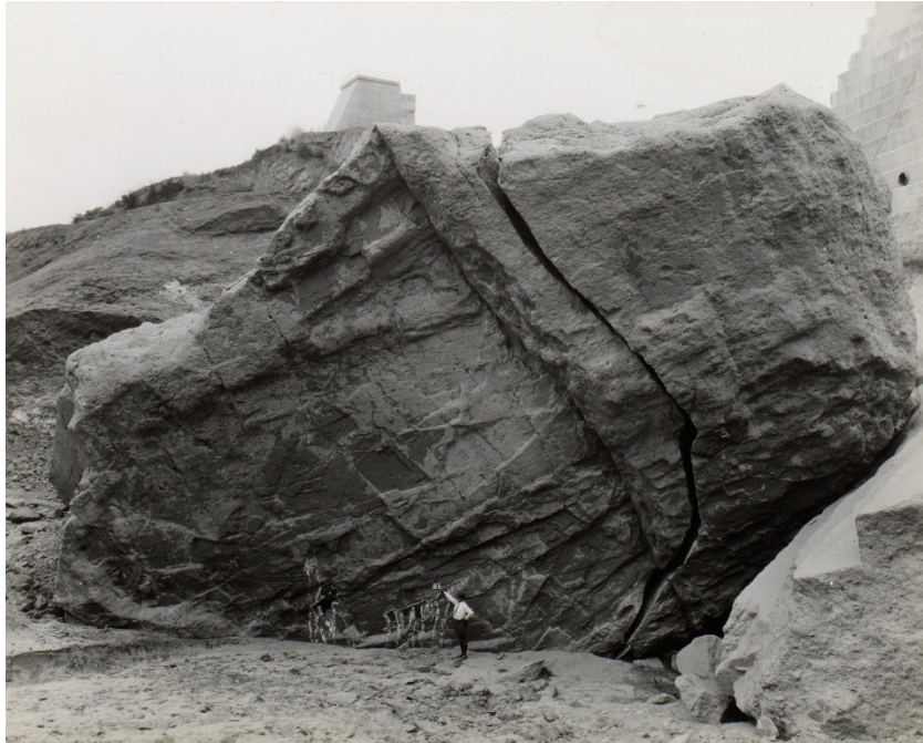
Figure 6. Upturned base of block #7, from the crest of the dam’s left abutment. The open fissure is transverse shrinkage crack #4, shown in the lower half of Figure 1 (Mayberry et al., 1928).
