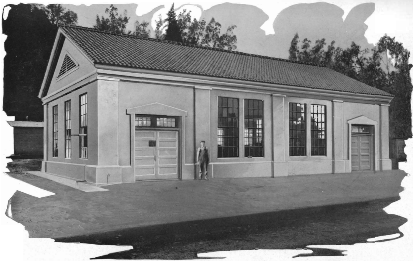
EXTERIOR - RIVERSIDE PUMPING PLANT. - JUNE 1923
