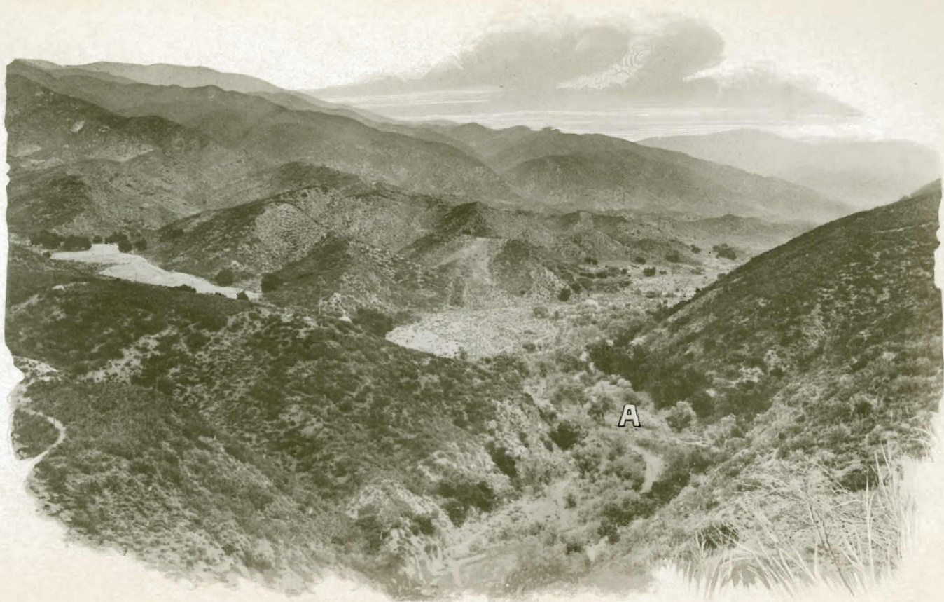
SAN FRANCISQUITO CANYON, SHOWING PROPOSED DAM SITE AND PORTION OF RESERVOIR. ("A" SHOWS APPROXIMATE LOCATION OF DAM.)
