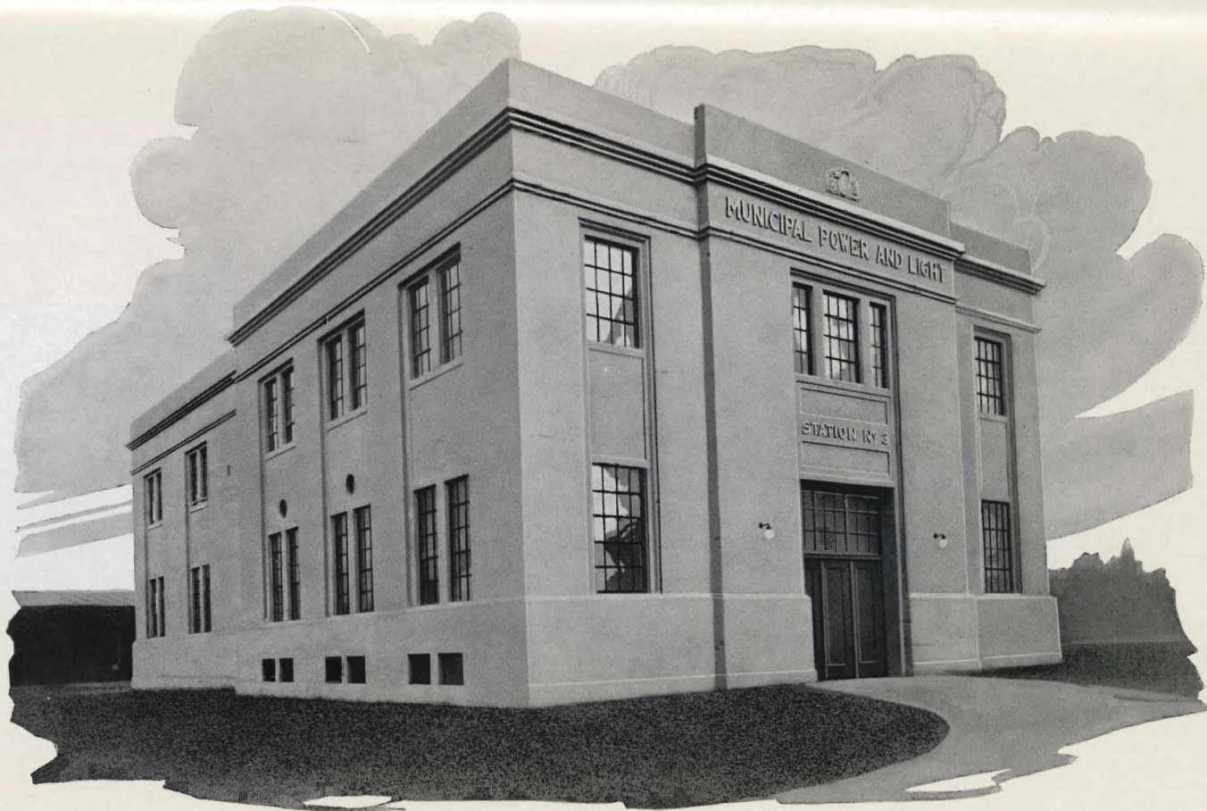
DISTRIBUTION STATION NO. 3, HARBOR BOULEVARD AND REGAN STREET, SAN PEDRO DISTRICT
