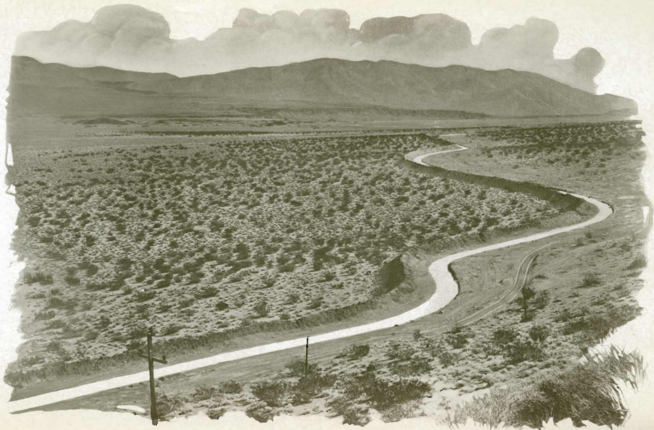
COVERED CONDUIT. FREEMAN DIVISION, LOS ANGELES AQUEDUCT.
