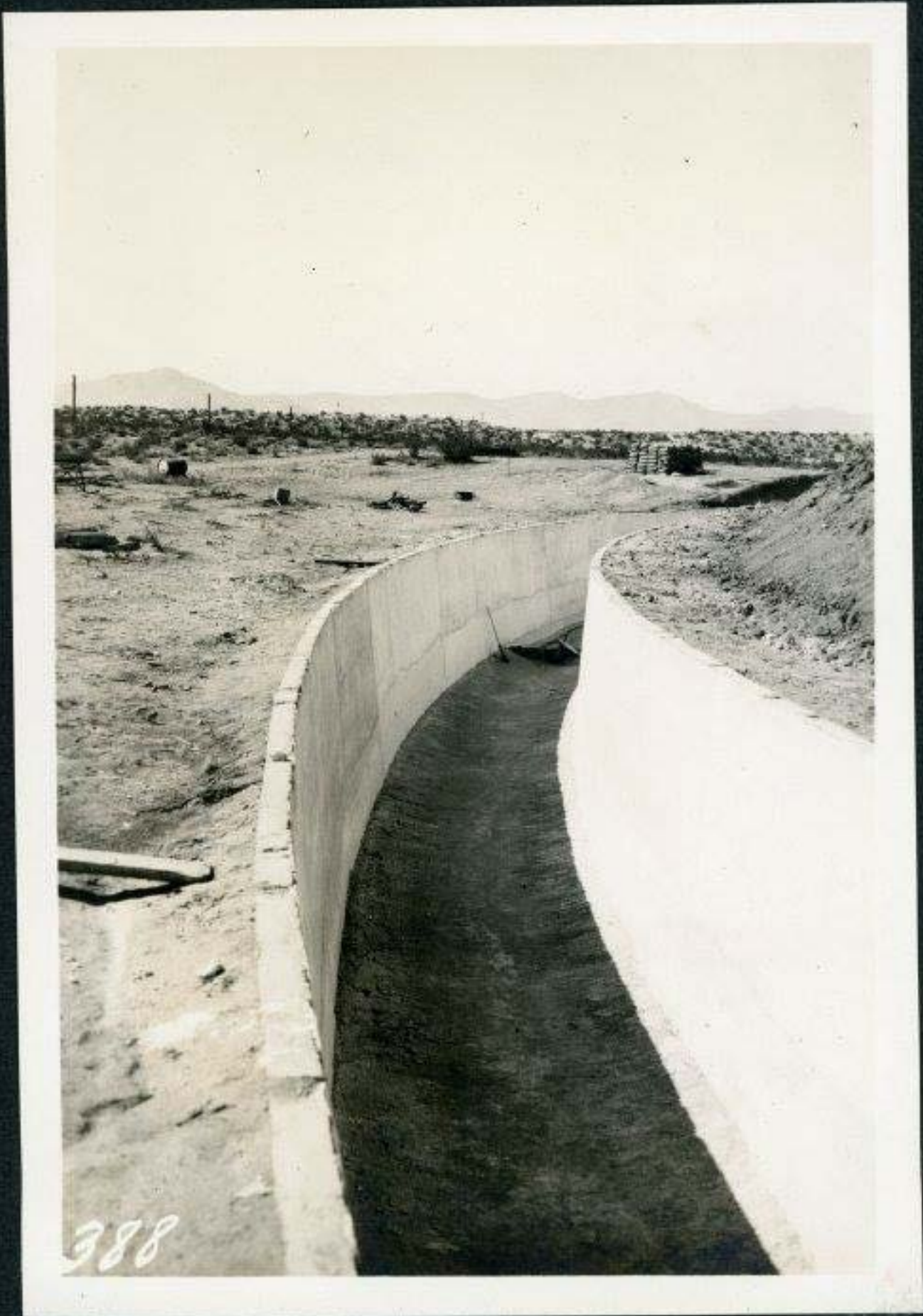
4. • Aqueduct in the Red Rock Country • • lined & ready for Cover •
