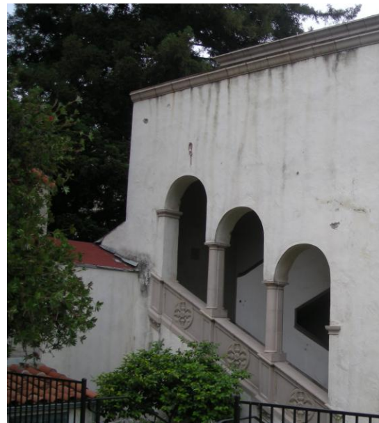
Staircase of West Wing with Classical cast stone floral ornamentation. July 9, 2012.
