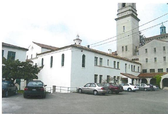
Service Wing, showing arched windows of small chapel, facing southwest. 2009, Courtesy of A. C. Cole, Historic Structure Report.
