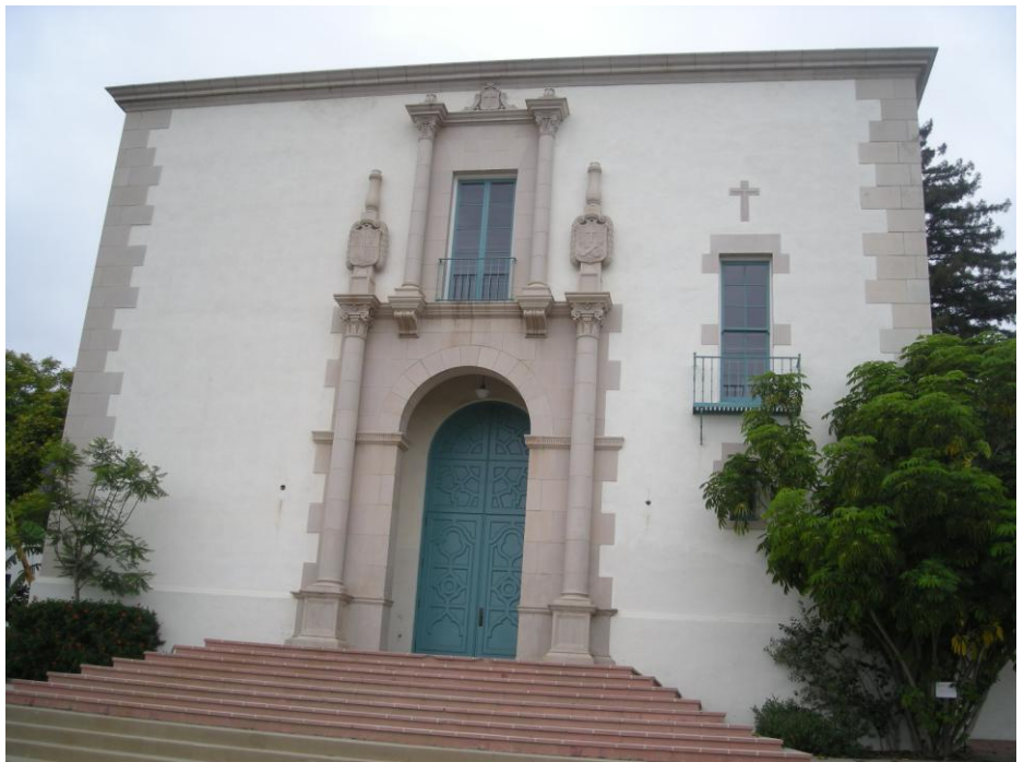
West Wing added in 1923. July 9, 2012.
