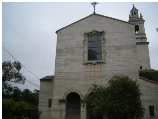
Front Elevation of St. Anthony's Romanesque Chapel. July 9, 2012.
