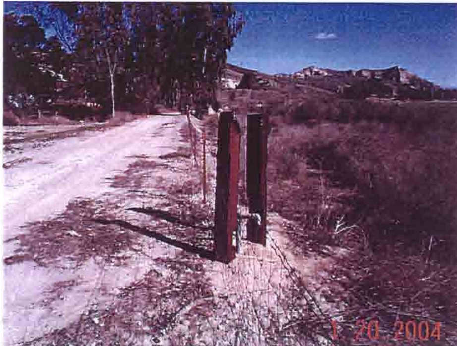
8. Vent pipe for oil pipeline.
