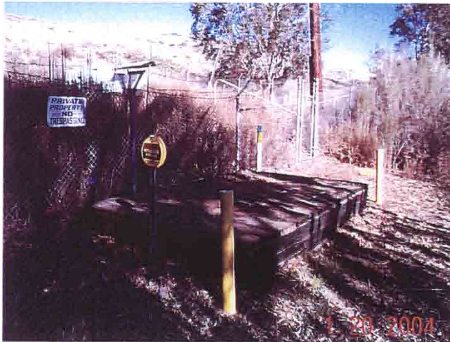
7. Access vault for Shell Oil pipeline.
