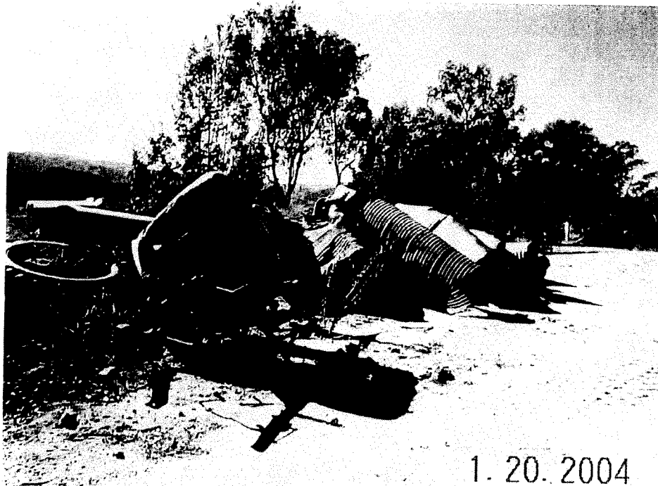
13. Metal debris in debris pile along northern property boundary.
