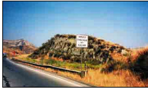
View Obstruction to be Removed by Project Improvements
