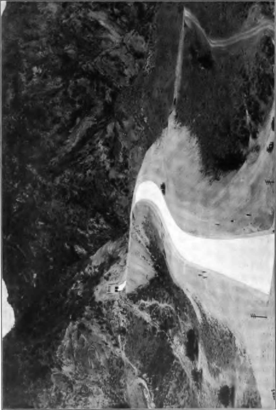
EXIT OF TUNNEL NO. 108, TERMINUS OF THE LOS ANGELES AQUEDUCT, SHOWING AERATING CASCADE
