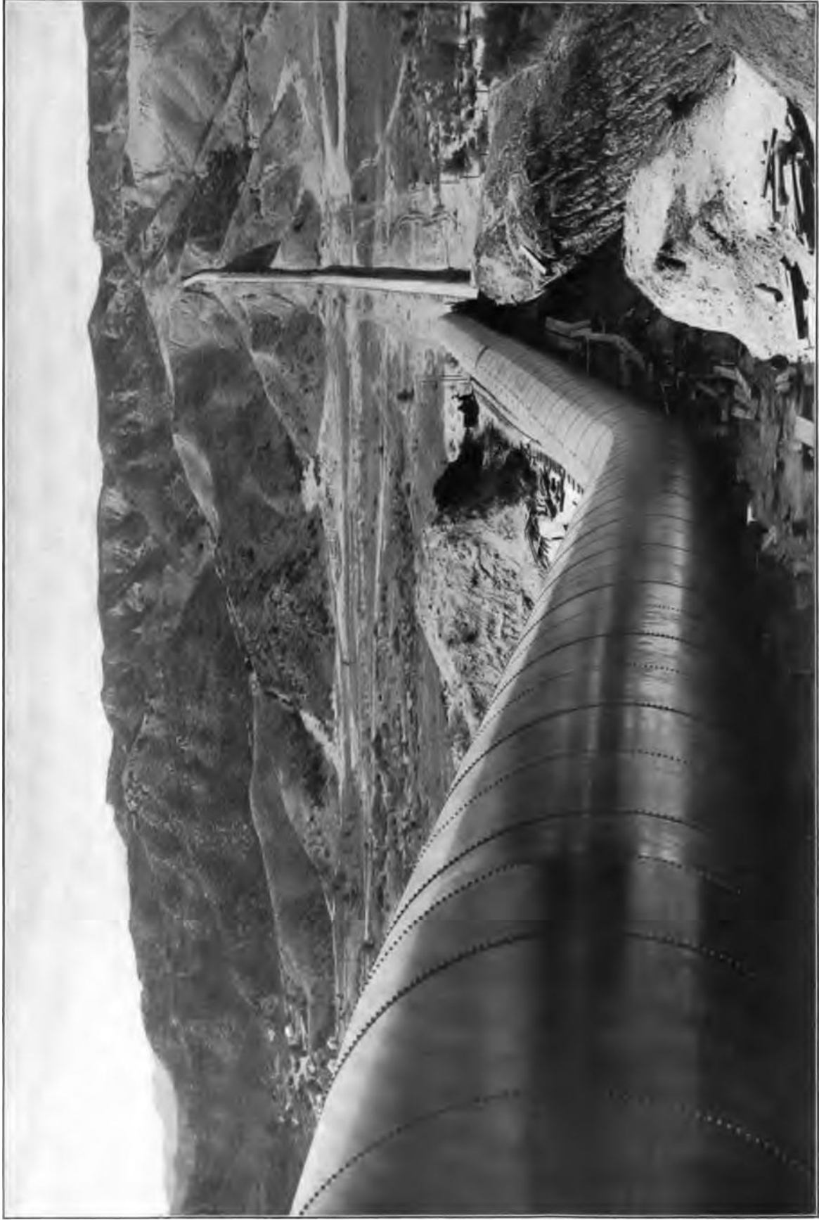
Deadman Siphon Looking Due North, Showing Pipe Before Concrete Piers Were Placed. North End of Steel Pipe Connected with Concrete Pipe which Follows Windings of the Crest of Hill
