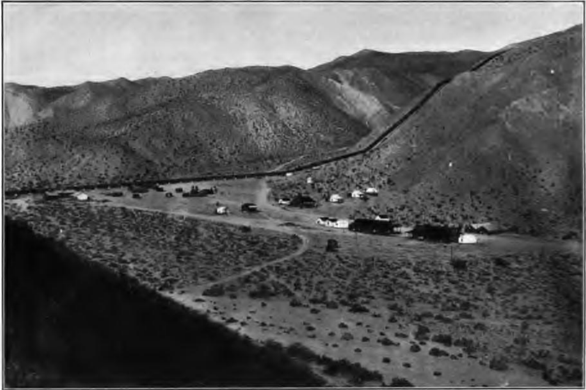
NORTH END OF PINE CANYON SIPHON
