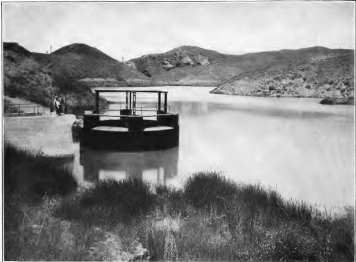
DRY CANYON RESERVOIR, SHOWING FLOATING WEIR
