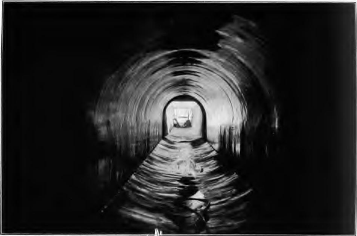
A Lined Tunnel in the Saugus Division
