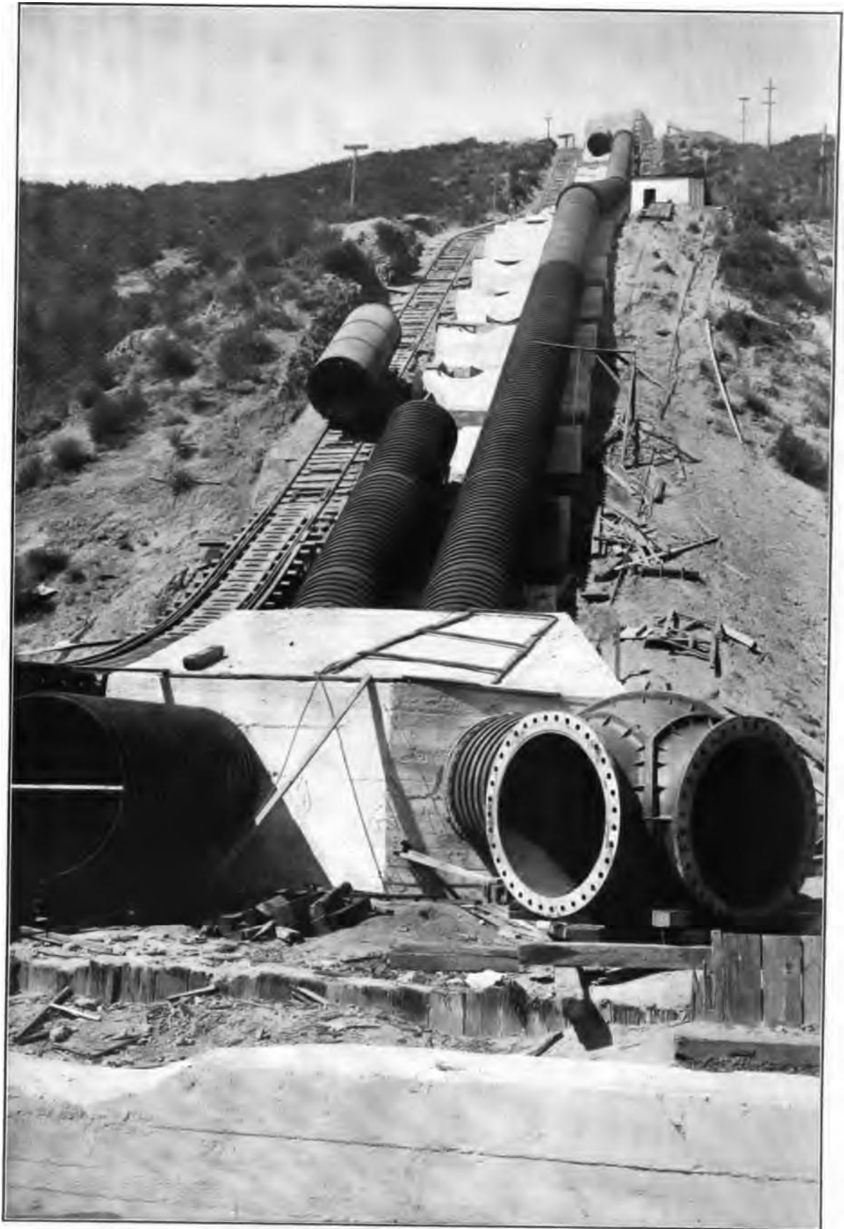
PART OF PENSTOCK OF POWER PLANT NO. 1
