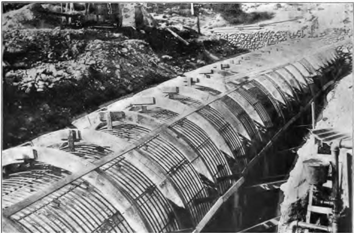
Concrete Siphon in Whitney Canyon. Photograph shows wooden forms. These were supplanted on other concrete siphons by steel forms
