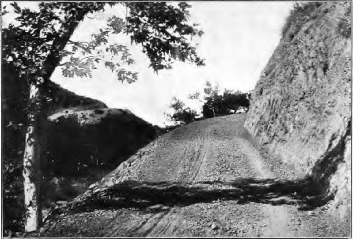
A CONSTRUCTION ROAD IN SAN FRANCISQUITO CANYON
