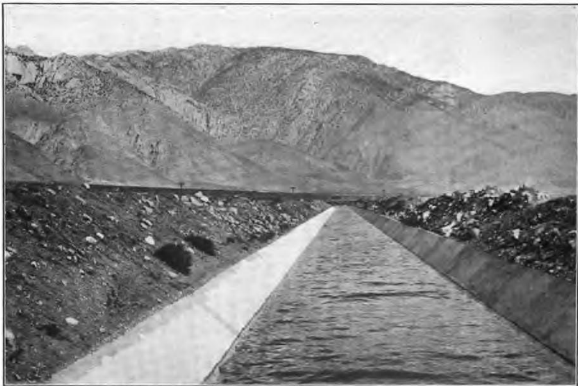
OPEN LINED CANAL IN OLANCHA DIVISION
