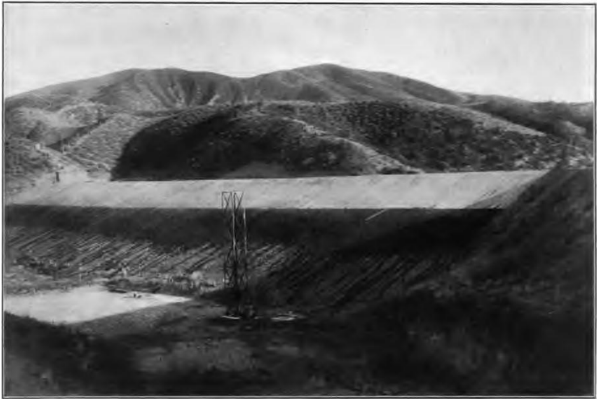
UPSTREAM FACE OF CANYON DAM
