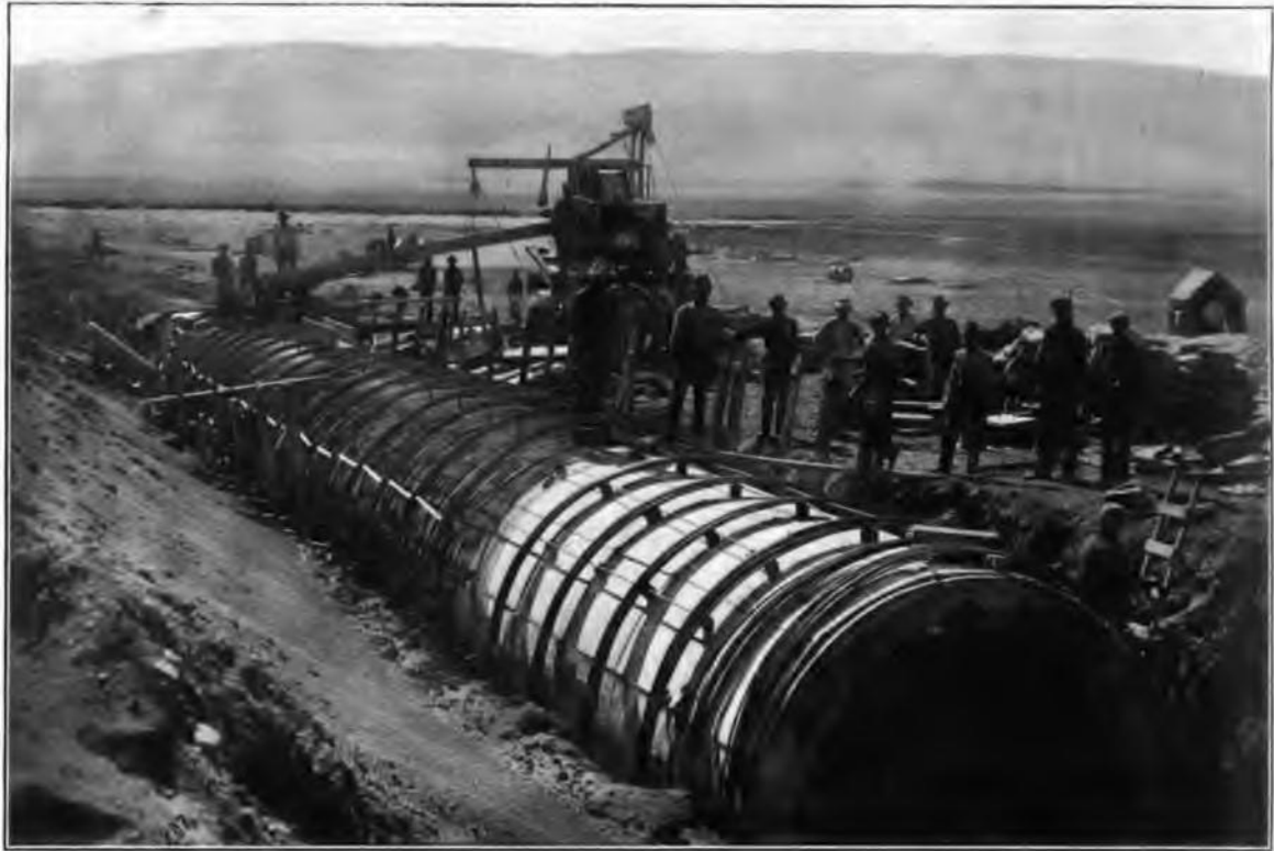
Forms for Concrete Portion of Antelope Valley Siphon
