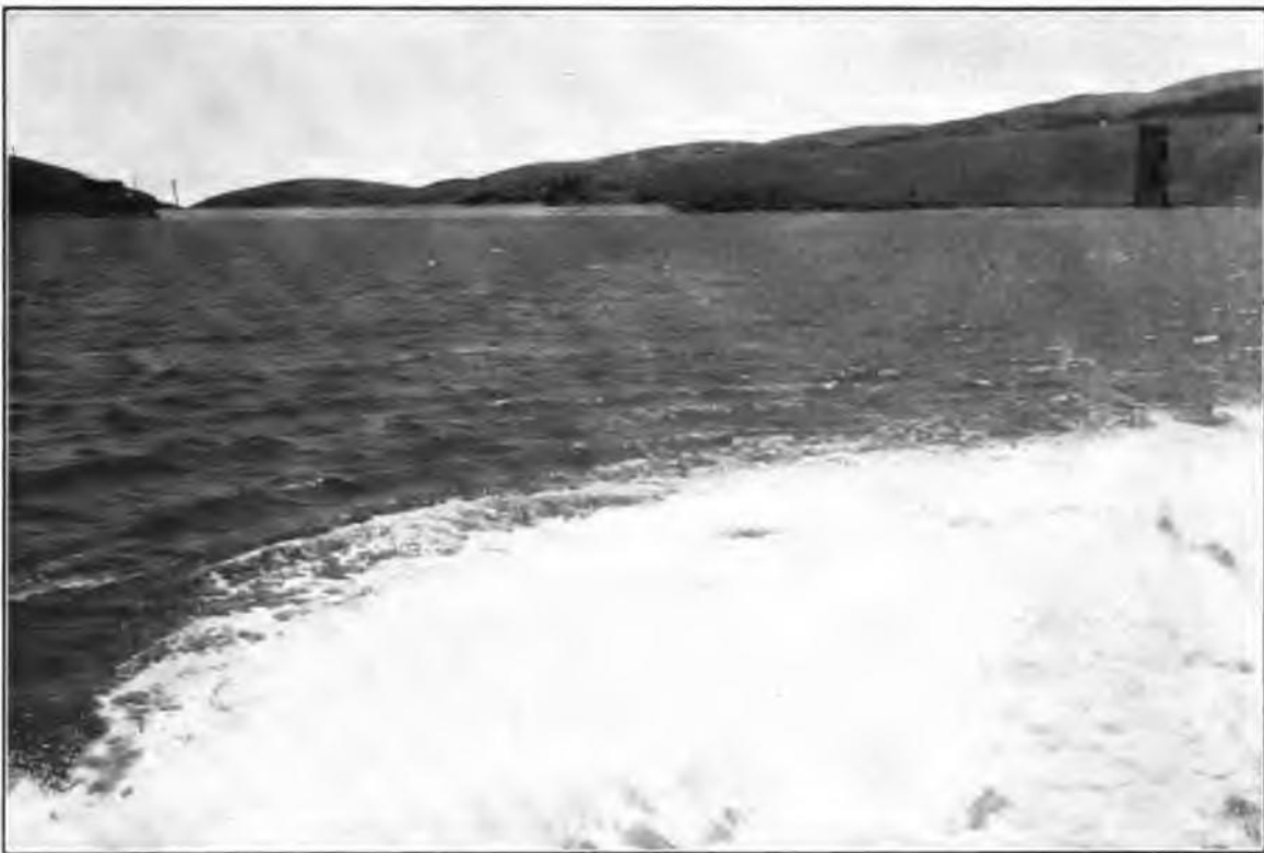
FAIRMONT RESERVOIR, LOOKING SOUTH FROM INTAKE
