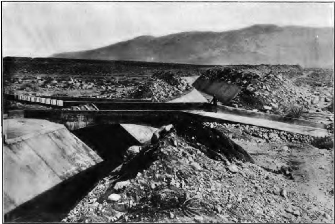
COTTONWOOD CREEK CROSSING THE AQUEDUCT
