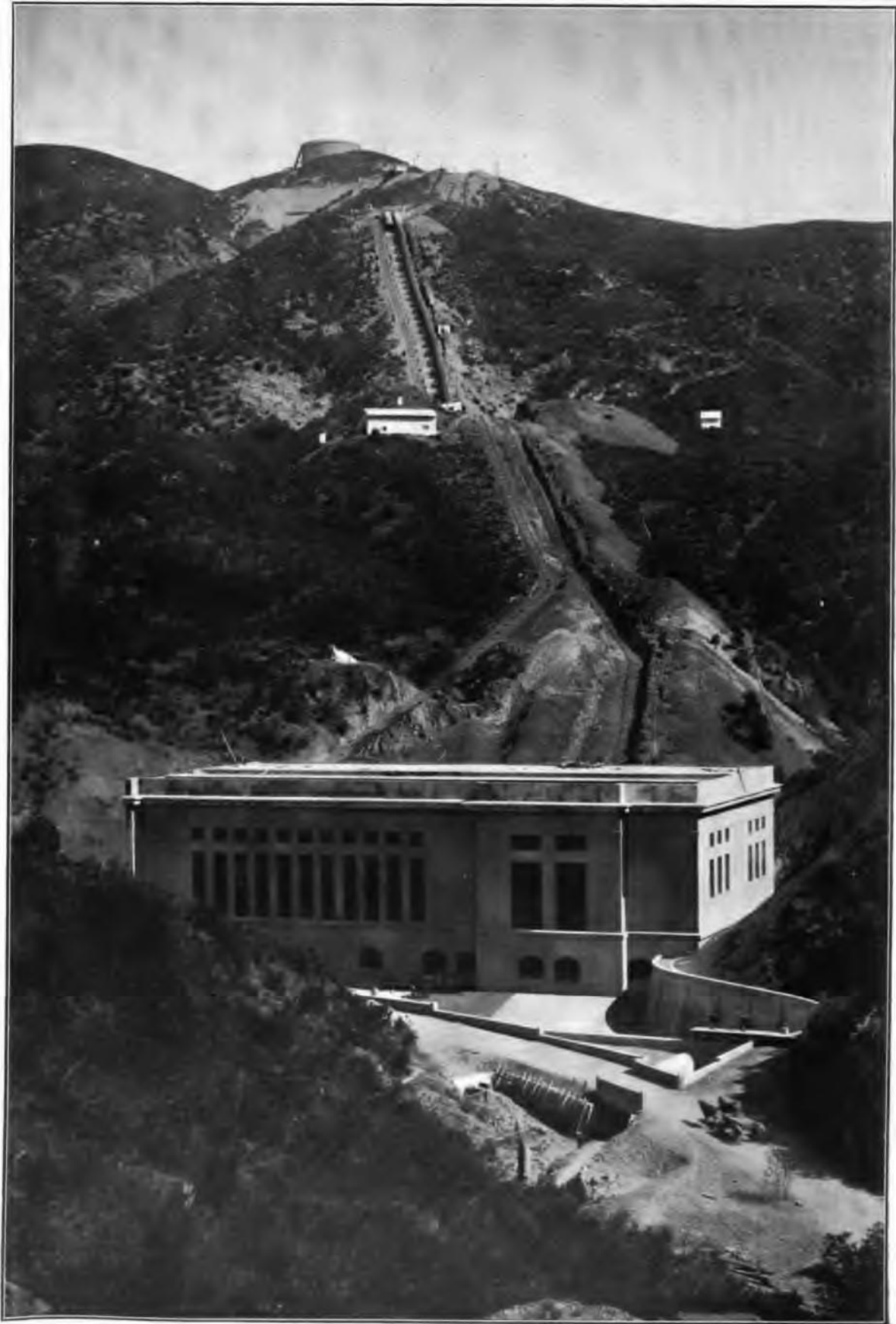
POWER PLANT NO. 1, SAN FRANCISQUITO CANYON
