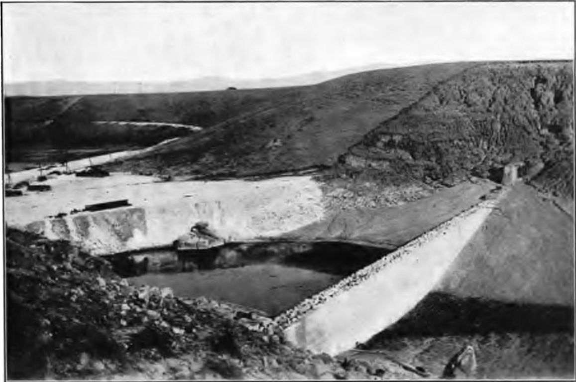
CORE WALL OF FAIRMONT DAM (Unfinished)
