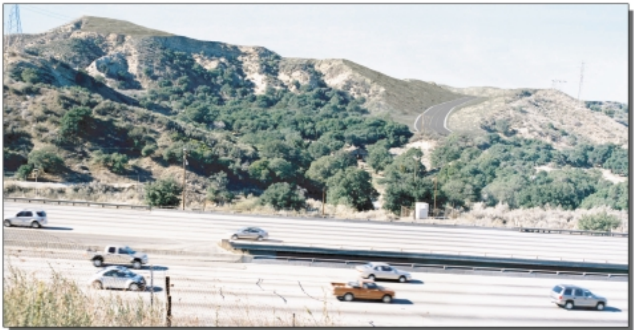
Post-project view from the same location. The roadway that can be seen is "C" Street.
