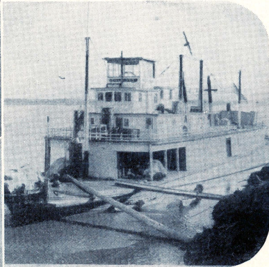
(Left) The first steel oil tanker built and operated on the Pacific Coast and the second built in the United States. It was launched by the Pacific Coast Oil Co. in 1895, and was named the "George Loomis" in honor of the company's second president. The oil tanker's capacity was 6500 barrels
