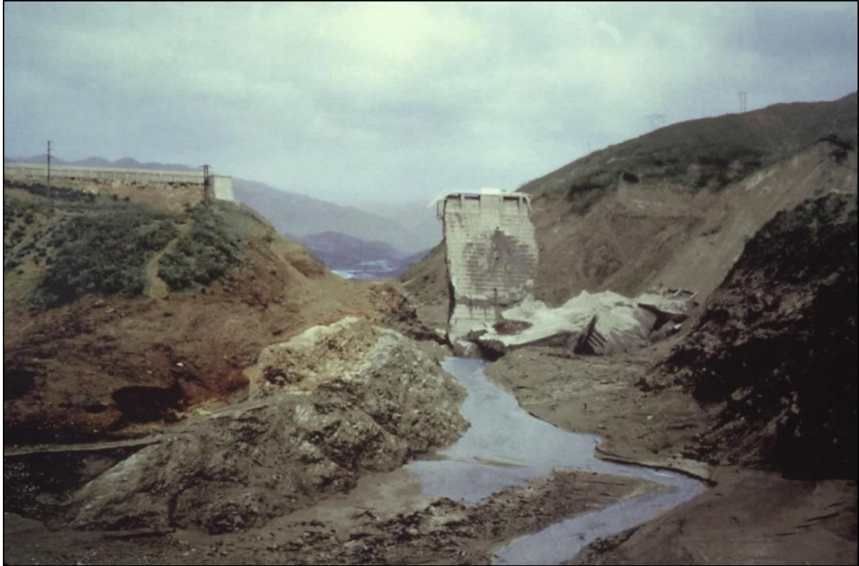
FIGURE 5.2 Upstream view of the remains of the St. Francis Dam, March 1928, illustrating the “tombstone” (C.H Lee Collection, U.C. Water Resources Center Archives, Berkeley, colorized by P. Horton).
