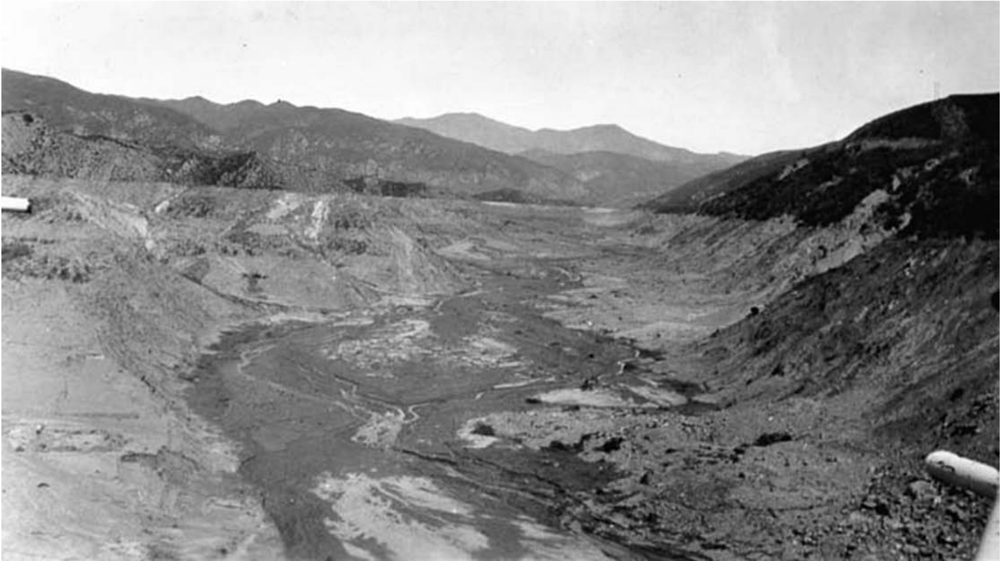
View from the top of the St. Francis Dam, looking north where the reservoir was located. The point between light and dark in the photo was the water line of the reservoir just before the dam failed on March 12-13, 1928.
