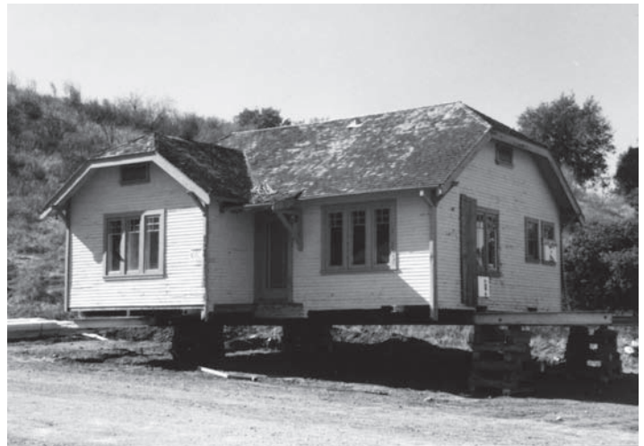
The Edison House arrives at Heritage Junction Historic Park - January 1989
