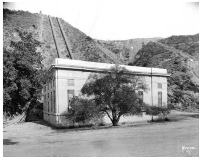
Power House No. 2, just below the dam, as it appeared in January 1928, two months before the disaster. The 41,800-hp power plant was located six miles below Power House No. 1 (which survived, since it was above the dam).
