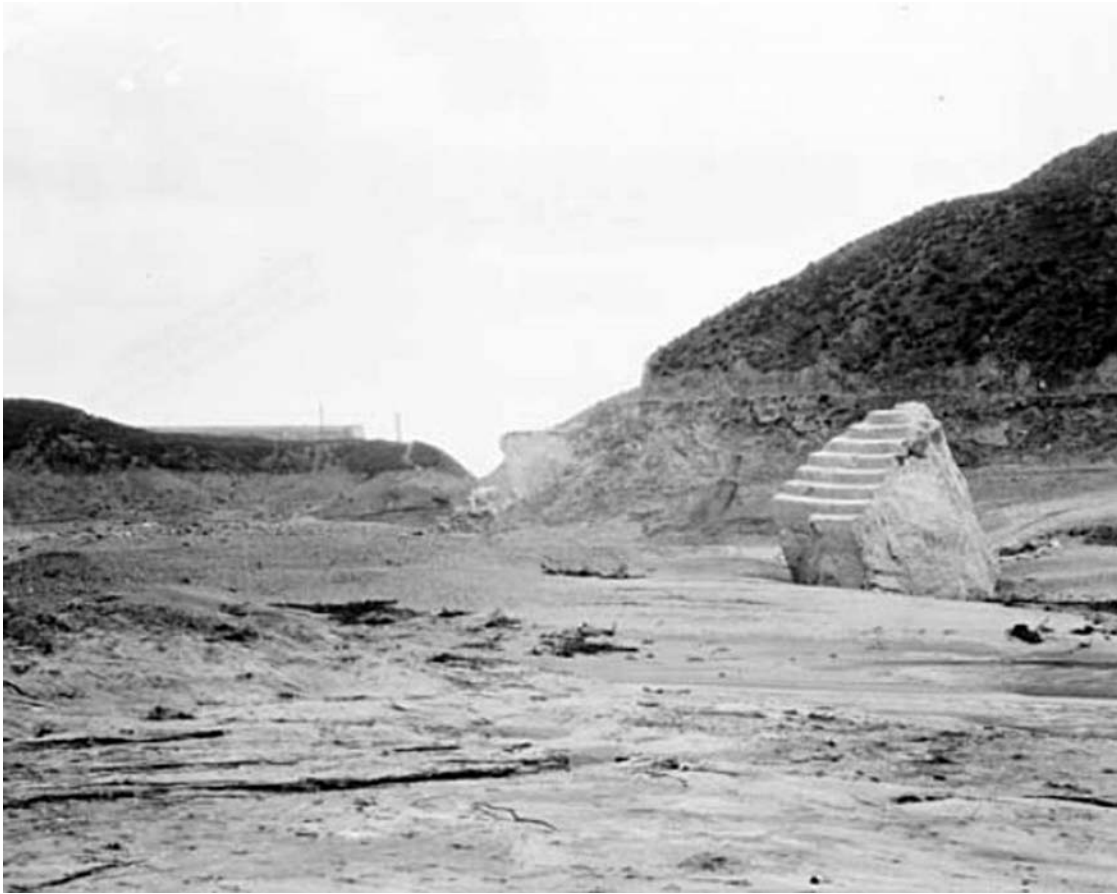
The force of the water forced this large concrete block downriver
