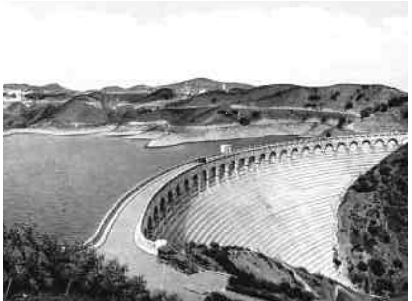
Mulholland Dam in the Hollywood Hills, a few miles west of downtown Los Angeles. Completed in 1924, Mulholland Dam (also identified at times as Weid Canyon Dam or Hollywood Dam) was the first concrete gravity structure built by Los Angeles under William Mulholland’s authority. Work on St. Francis Dam commenced soon after completion of Mulholland Dam. Testimony at the coroner’s inquest revealed that the design of the latter, with its stepped downstream face, served as a model for St. Francis Dam.
