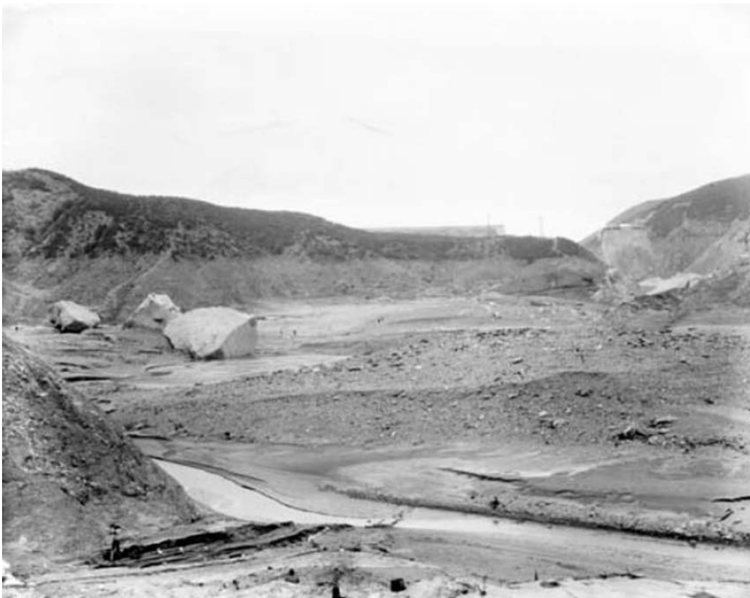
Large concrete blocks have been washed downriver from their original location at the right of this photograph following the collapse. Some of the “specks” in this photo are people examining the wreckage.
