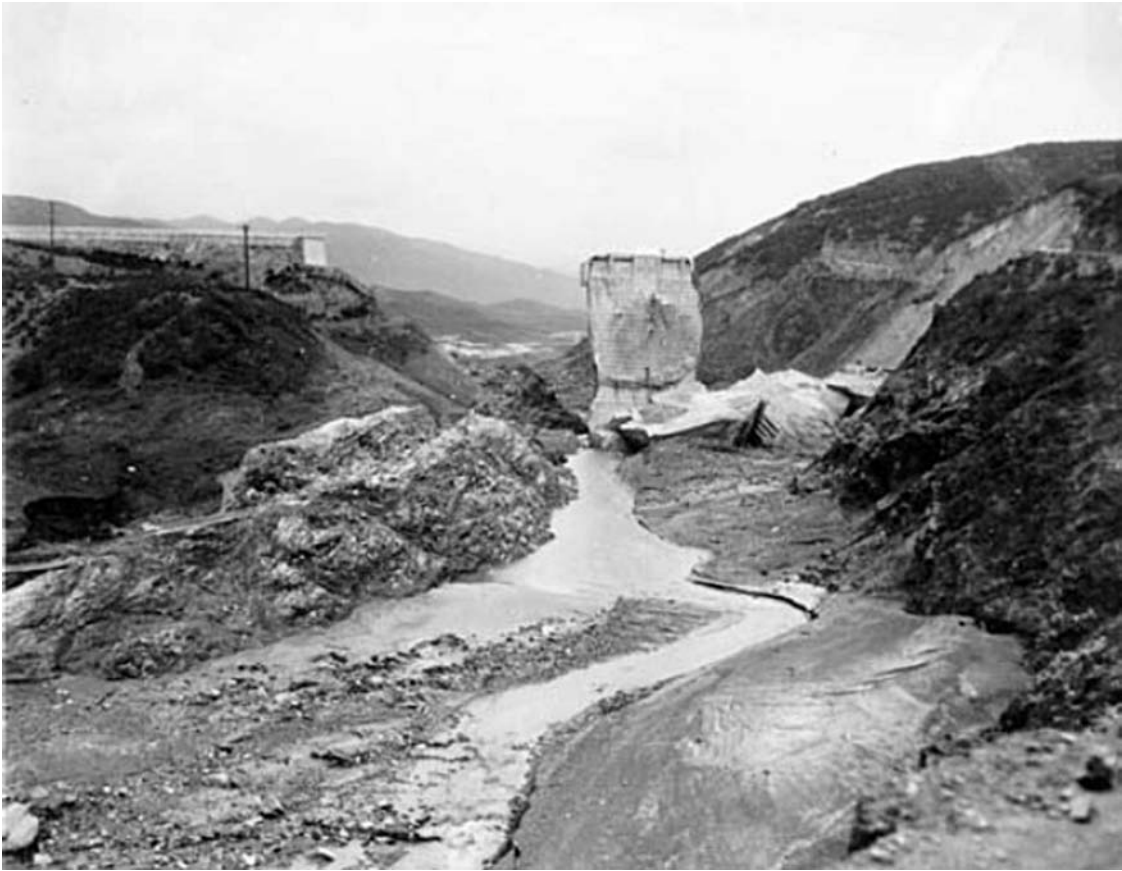
The torrent has slowed to a trickle following the March 12-13, 1928 failure of the St. Francis Dam in San Francisquito Canyon.
