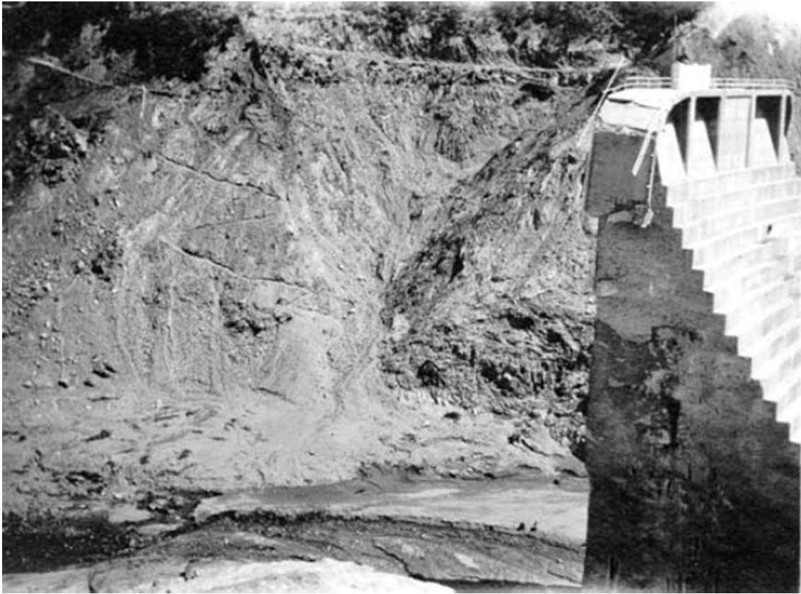
The “tombstone” and the hillside to the east behind it, showing the landslide area with the old road at top.
