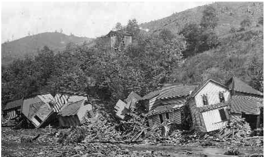
TOP: Aftermath of the dam failure at Austin, Pennsylvania, on September 30, 1911. After visiting the Austin site in October 1911, John R. Freeman and Arthur Powell Davis—two of Mulholland's engineering colleagues who had recently served with him on a consulting board for the Great Western Power Company—recognized the role of uplift in the Austin collapse.
