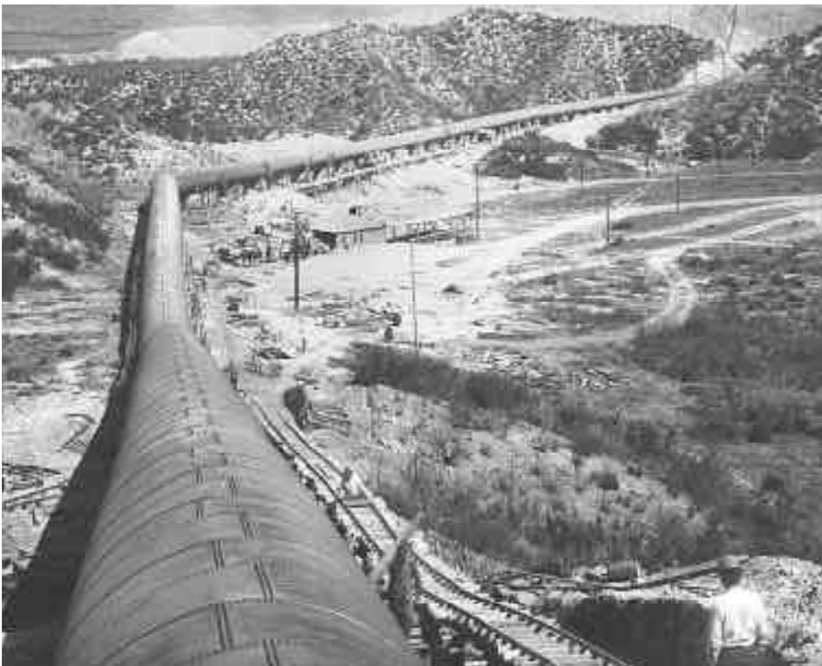
LEFT: Extending across the barren expanse of the western Mojave Desert, the aqueduct carries water over 200 miles from the Owens River Valley to the city. This section is the Soledad siphon near Saugus, about ten miles south of San Francisquito Canyon.
