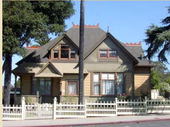
The front facade of the Shipsey House after restoration
