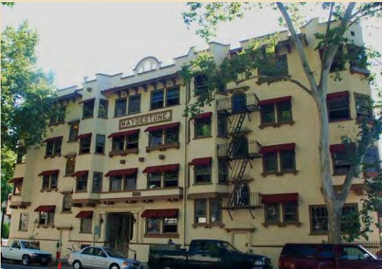
The Maydestone is a 1912 Mission Revival style apartment building.
