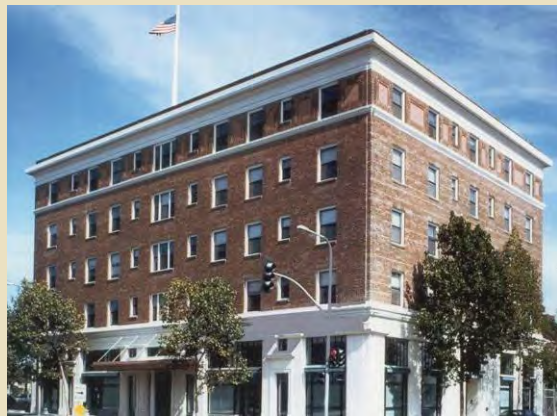
The Carquinez Hotel was a Federal Tax Credit project now with low-income senior housing and commercial space on the first floor.
