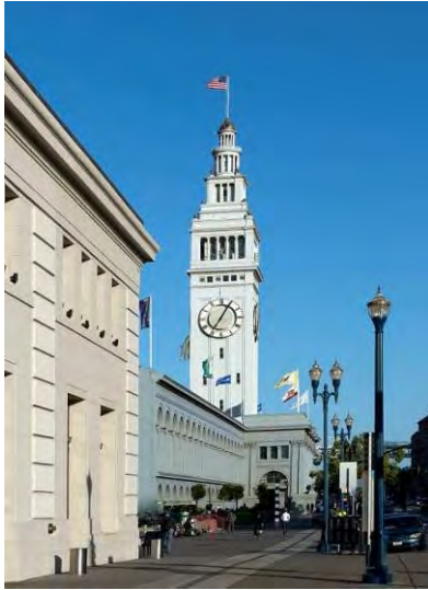
The owners of the Ferry Building made use of Federal Rehabilitation Tax Credits as part of their very successful adaptive reuse of this well-known San Francisco landmark. (Photo from the Carol M. Highsmith Archive, Library of Congress, Prints and Photographs Division)
