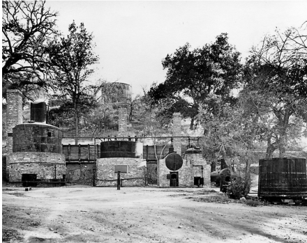
From left to right: still 4, still 3, stills 1&2, boiler, "residium" tank (SCVHS)
