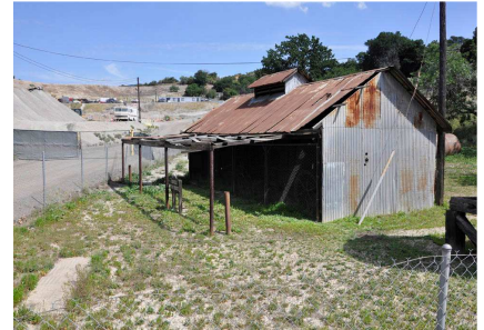
Existing Pump House – May 2016 (Knapp)
