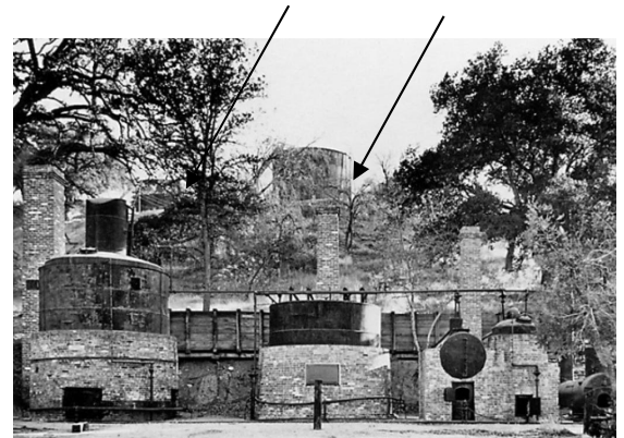
Two storage tanks are visible through the trees on the hillside above the stills in this photo taken after the 1930 restoration. (Photo courtesy SCVHC.)
