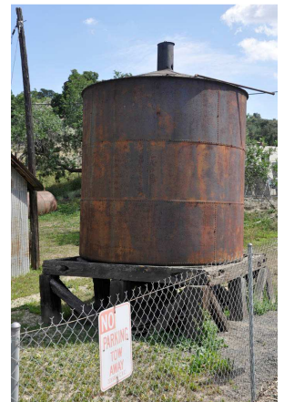
Acid Wash Tank, 2016 (Knapp)
