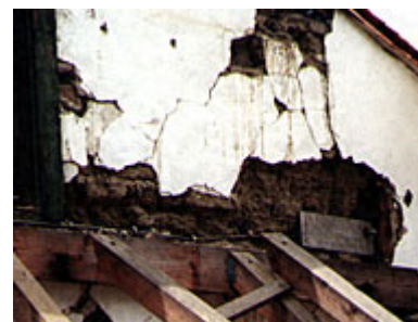
A detail of the east gable during
