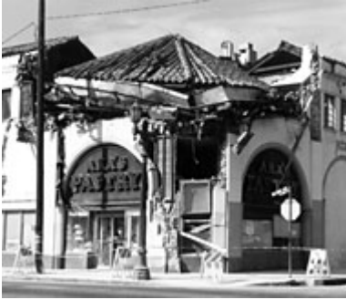
The Ara's Pastry building, located in Hollywood. Built around 1925, the structure has received grants for technical assistance, repair, and restoration, and work is under way. Photo: Lisa Snyder for the Los Angeles Conservancy.
