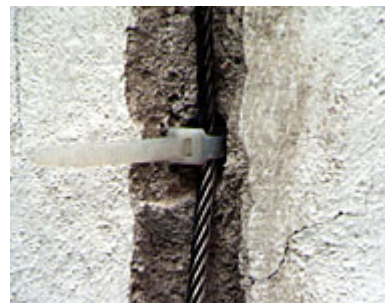
A detail of a steel cable and nylon tie.
