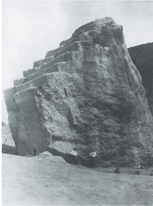
Figure 37. Close-up view of Block 16 (State designation) or 44 (BWWS designation), at 10,000 tons, the largest of the dam's displaced blocks. It was found about 1,500 feet downstream of the dam. The only plausible mechanism by which such a large block could be hydraulically transported would be by saltation in a dense slurry, akin to a massive debris flow. Photo from the Lee Collection, U.C. Water Resources Center Archives.
