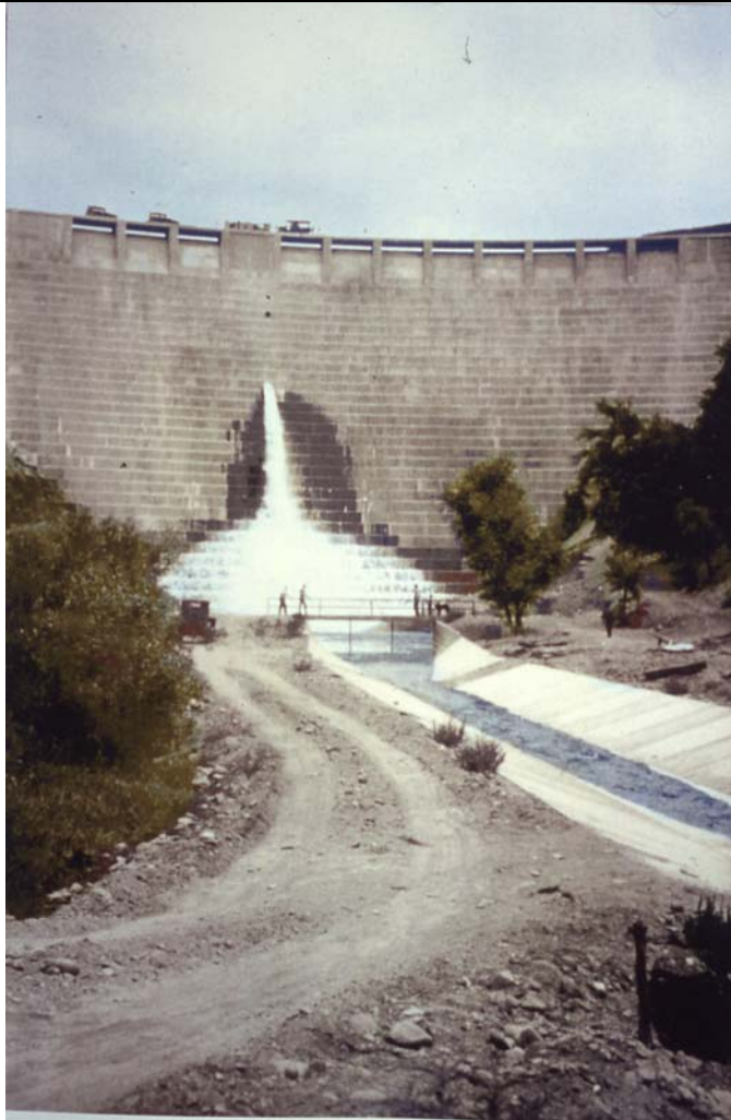
Figure 12. Frontal elevation view of St. Francis Dam, believed to be taken the day of dedication, in May 1926. Note the eleven crest spillway bays, each only 18 inches high, and the concrete-lined trapezoidal channel in foreground, which ran 7,300 feet downstream, to Powerhouse 2. Image colorized by Pony Horton.
