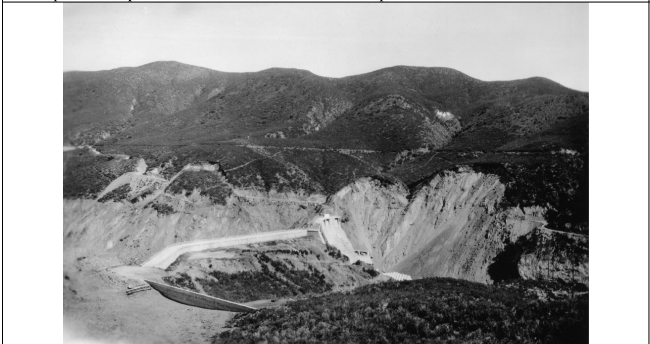
Figure 10 (lower). Same view taken after the failure. Note the prominent topographic bench in the Sierra Pelona escarpment, caused by massive landslipping. The east abutment slide is at right center. Another slump is obvious at left center, which dropped the old San Francisquito Cyn. Rd. about 50 feet (profiled in Fig. 45). From La Rue Collection at the Huntington Library.
