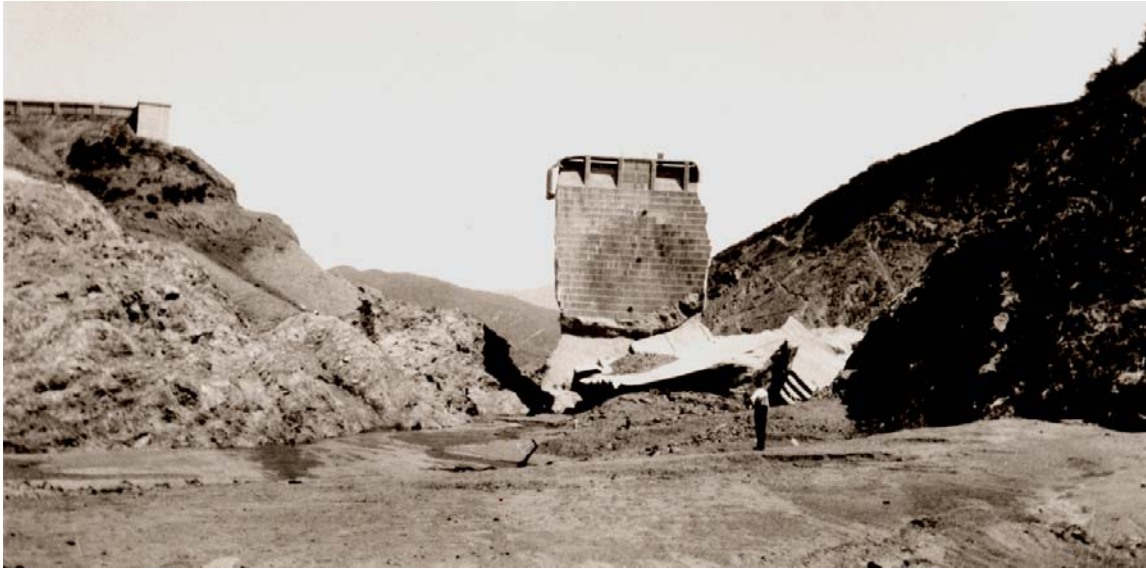
Figure 59. View looking upstream at the imposing monolith of Block 1. As in the previous photos, the gap between Block 5 and the chatter mark cut into Block 1 is noticeable, as is the clean character of the right abutment, swept clean of all debris in the later stages of the failure. Photo from the W.L. Huber Collection of the U.C. Water Resources Center Archives.
