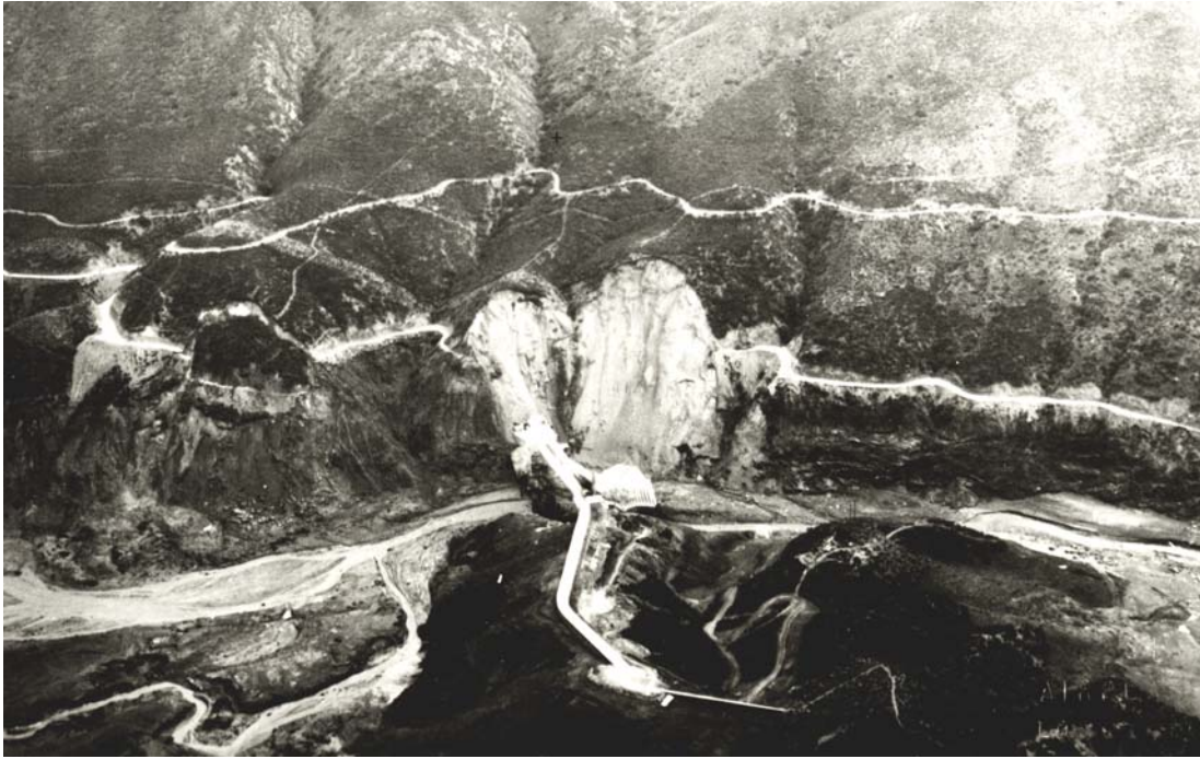
Figure 28. Aerial oblique view of the dam site by Spence Aerial Surveys the morning after the failure. Note the position of the east abutment landslide and old San Francisquito Canyon Road with respect to the dam (from the UCLA Spence Photo Collection).
