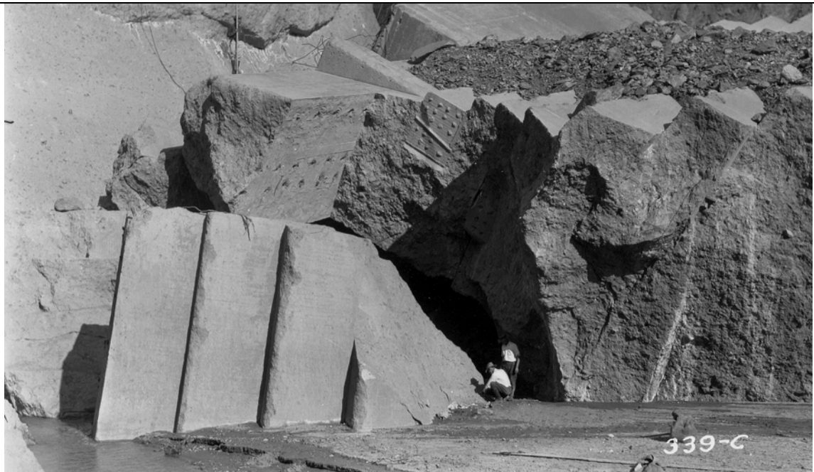
Figure 58. State survey party examining Block 6, which fell off of Block 5. Note the schist detritus infilling the 5 foot high steps of Block 5, 25 to 30 feet above the channel in foreground. Photo by H. Wildey, from author's collection.
