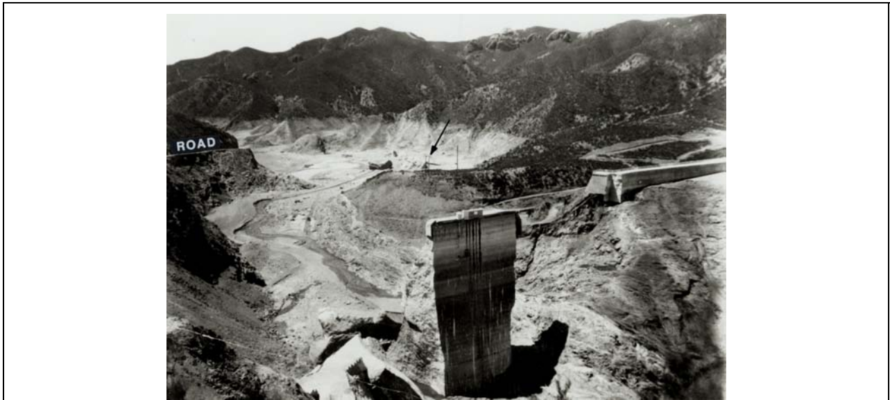
Figure 14. Downstream view of the dam site after the failure, showing location of the SCE 70 Kv Borel Power Line poles, about 60 feet above the high water mark on the right abutment, about 650 feet downstream of the dam. Photo from Ventura County Museum of History and Art.
