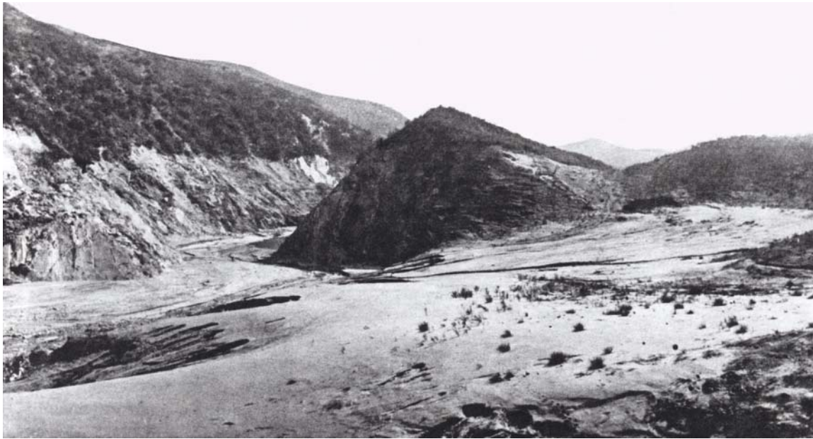
Figure 31. Downstream view of the silt blanket deposited by the flood, just above the first hairpin turn of San Francisquito Creek, about 1,000 feet upstream of Powerhouse 2 (taken from the 'C' in Canyon on Fig. 36). The flood detritus is predominately Pelona Schist, and the grain size distribution is quite uniform. At the peak of the outbreak flood, water spilled over the saddle at middle right (from the Huber Collection, U.C. Water Resources Archives).
