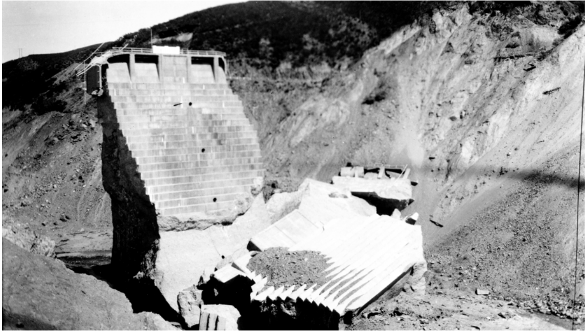
Figure 57. Upstream view of Block 5 sitting in front of Block 1 after the failure. Note the quantity of schist detritus sitting atop Block 5, testifying to its having been carried down slope in a slurry of disaggregated schist. Note the chatter marks on Block 1 cut by Block 5 and the latter's final resting position, about 30 feet lower. The material originally supporting Block 5 was likely swept away when the right abutment subsequently failed. Photo from the Lee collection, U.C. water Resources Center Archives.
