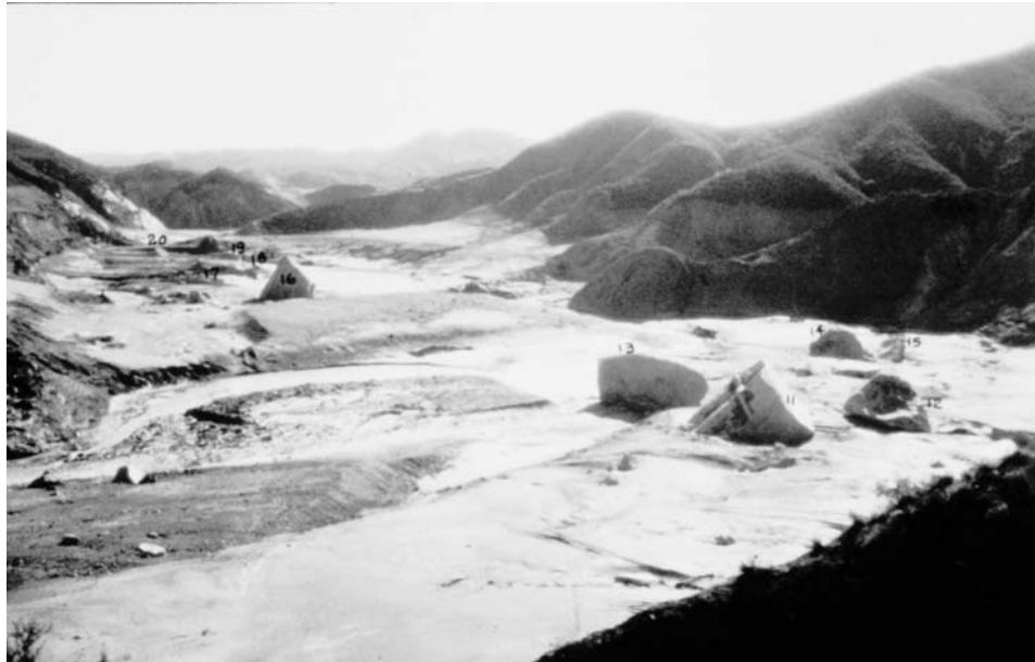
Figure 36. Displaced blocks of the dam, as viewed from a position about 1,000 feet downstream of the dam site. The block numbers written on the photo are those of the State Board of Inquiry (Fig. 38). Although Blocks 12 and 14 came from the base of the left abutment, they were situated between 22 and 26 feet higher than Block 16, seen further downstream and within the low flow channel.
