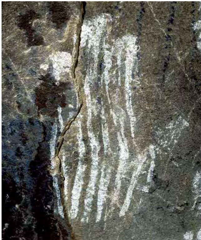
Figure 21. This is one of the clearer examples. Note the light scratched lines to the right of the hand, as well as over the bottom third. This is from vandalism. Note also the severe crack forming along the left side of the hand.
