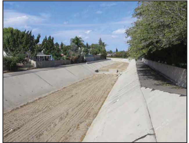
View 8: View from Wiley Canyon Road looking northwest along Pico Canyon Wash.
