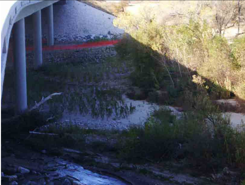
Photo 3. Upstream of I-5 Bridge at Santa Clara River Crossing
