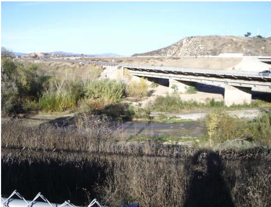
Photo 4. Santa Clara River downstream of the Old Rd. Bridge
