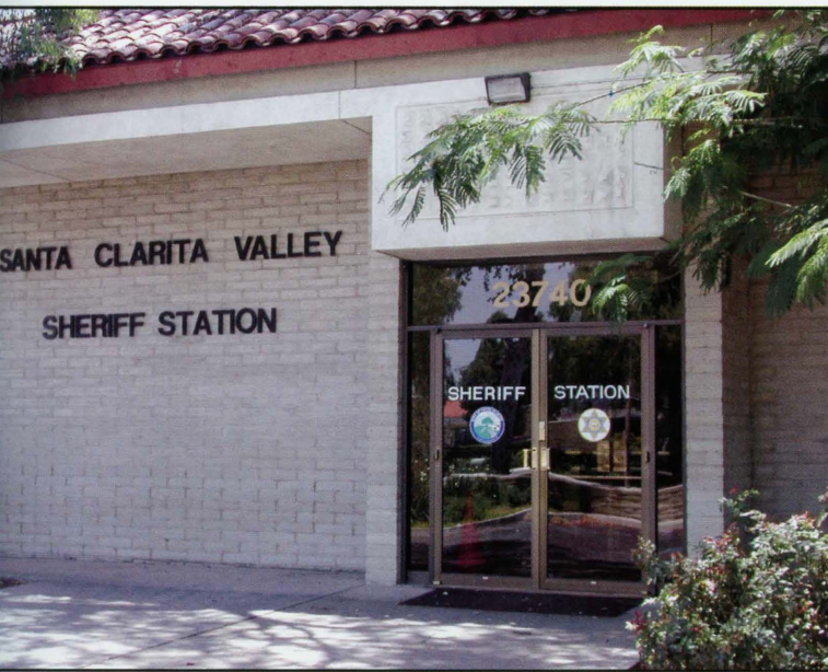
The Santa Clarita Valley Sheriff Station is home to the various specialty teams and deputies who provide law enforcement services to the residents of the Valley.
