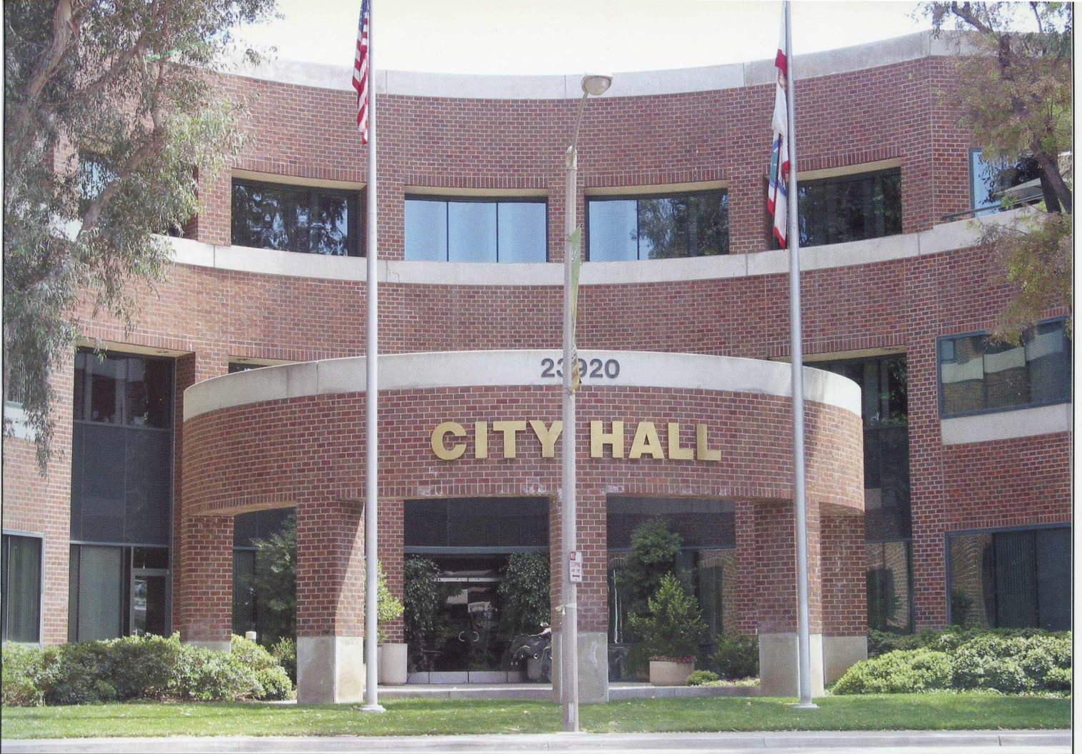
Above: Santa Clarita City Hall is located at 23920 Valencia Blvd. in Santa Clarita. This facility houses more than 250 city staff members.
