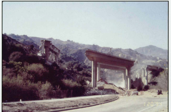
The earthquake caused millions of dollars in damage to local roads and freeways. Pictured here is the collapse of a bridge along Interstate 5 in the Santa Clarita Valley.
