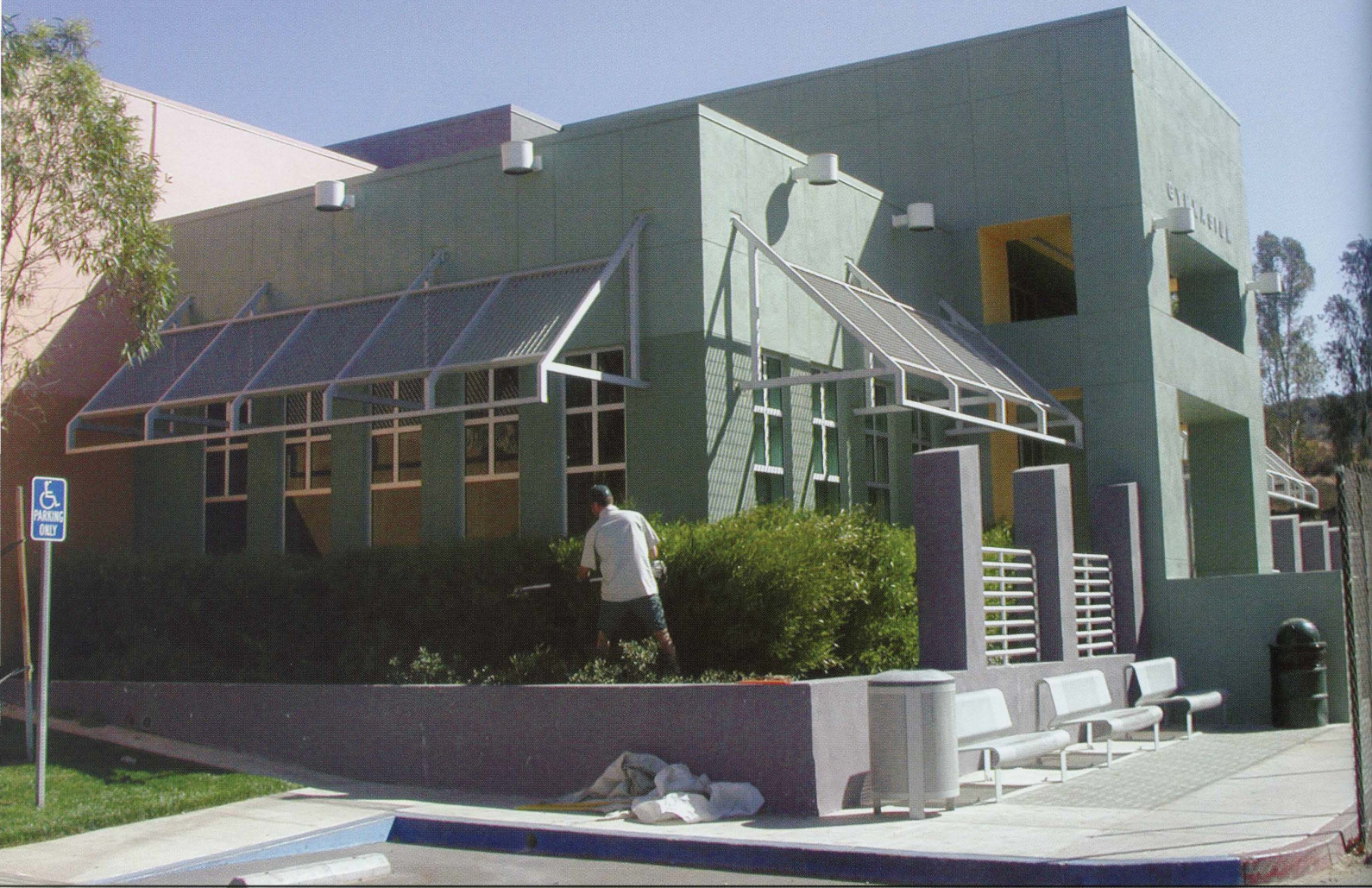
The Santa Clarita Activities Center is part of the 20-acre Santa Clarita Sports Complex and includes a performance area and a banquet room, as well as classrooms and offices.
