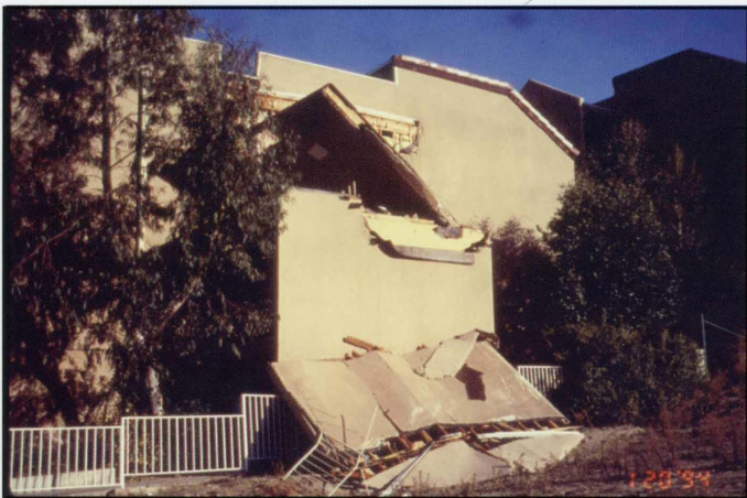
Buildings, homes, roads, walls and bridges collapsed as a result of the 1994 Northridge earthquake that rocked Santa Clarita Valley.
