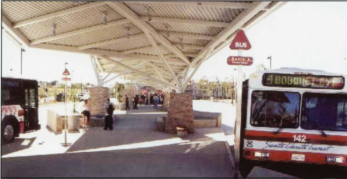
Santa Clarita Transit services the City's three Metrolink stations as well as the McBean Transfer Station.
