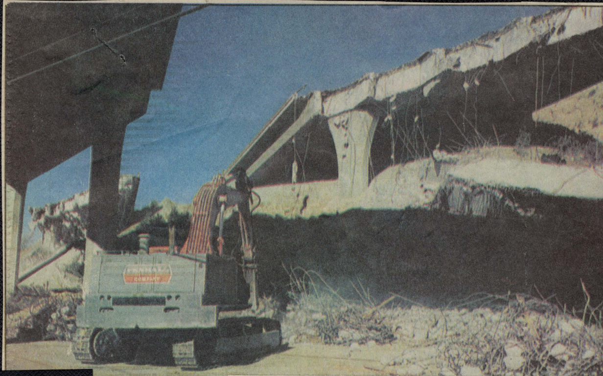
Workers continue to remove parts of the collapsed Antelope Valley Freeway connector ramp Friday. Detours around the severed junction are expected to be in place next week.
