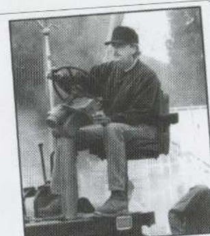
Vince Brutz operates the paving machine on March 3rd.
