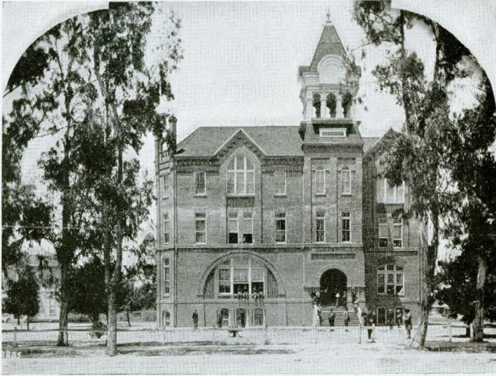
The start of the University of Southern California back in the eighties The University was founded in 1880
