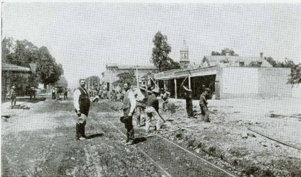
Double tracking the horse car line down Main Street in late seventies. Note spire of Santa Vibiana Cathedral still standing near Second Street.
