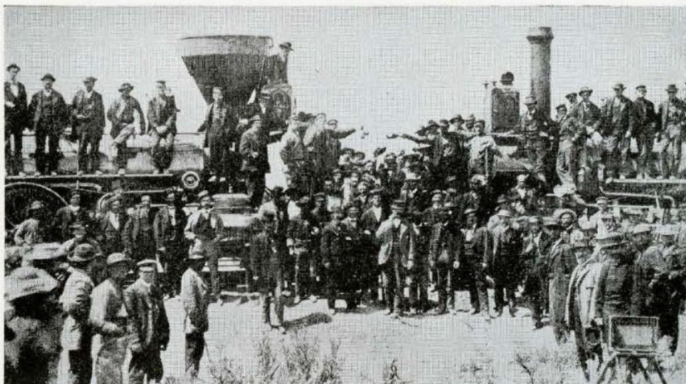
Union of the rails at Promontory, Utah, May 10, 1869 marking completion of America's first transcontinental railroad Seven years later this railroad reached Los Angeles
