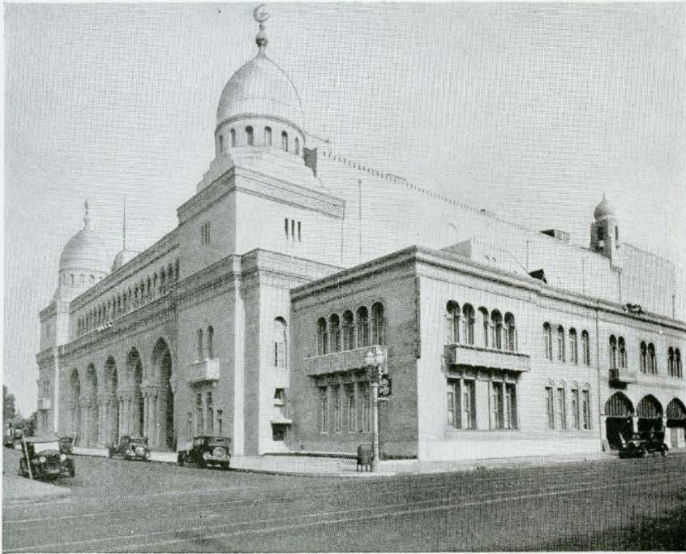
The new Shrine Auditorium
