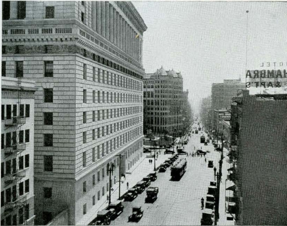
Looking down Broadway from above Temple, 1928 showing new Hall of Justice at left Compare with picture on page 52, taken from same spot
