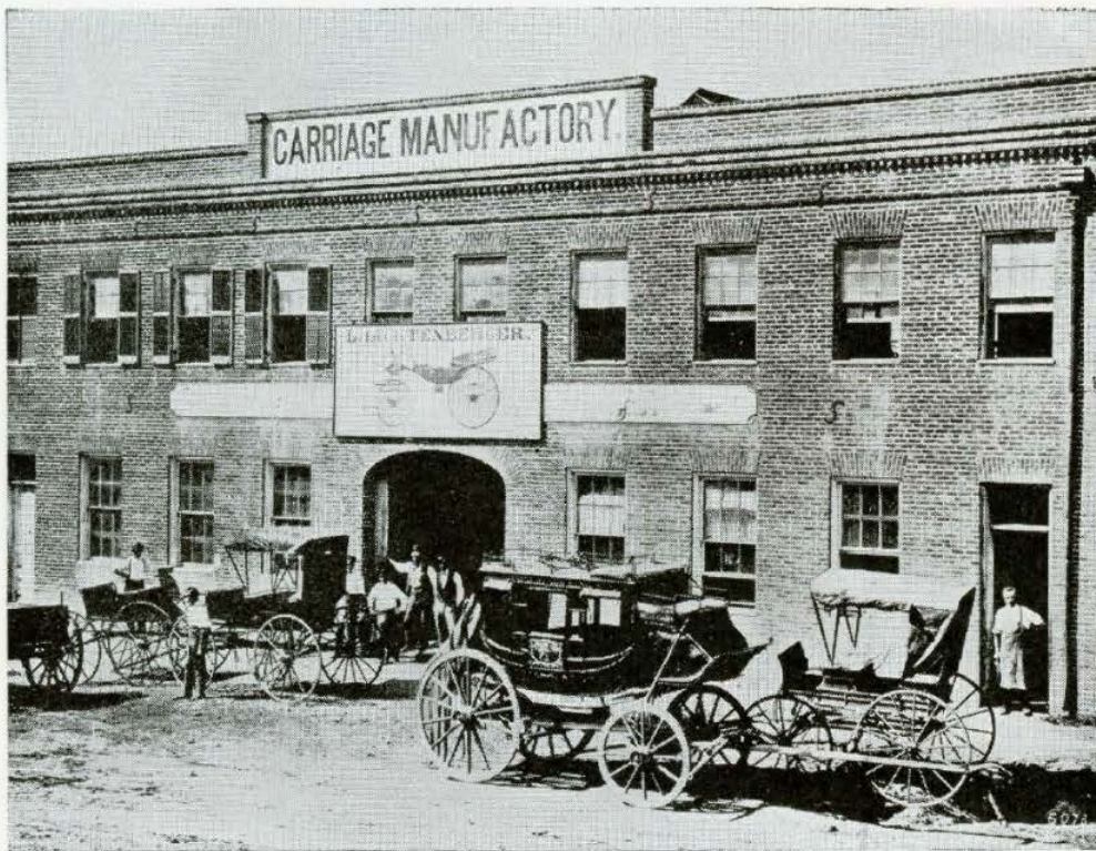
The Lichtenberger carriage factory was one of the city's largest industrial plants in the seventies
