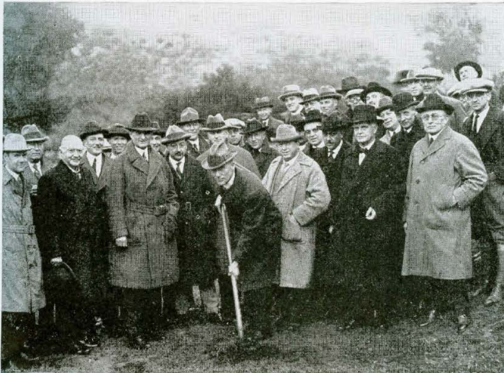
Mayor Cryer breaking ground for the Mulholland Highway in 1923
