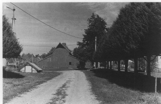
Figures 22 and 23: The plan for the Kehlbeck Farmstead, located in Cass County in Southeastern Nebraska, illustrates a well-planned, and aesthetically arranged general farm complex of the twentieth century. The farmstead is composed of 23 contributing and 5 non-contributing resources. Integrity was judged uniformly high because many character-defining resources were present and the visual and spatial relationships intact. Note the varied graphic techniques used to document a variety of fence types, and, the key to photographs illustrating the various landscape features and spatial relationships. The photograph above, labeled #3 on the farmstead, is looking north along the farm lane allée. (courtesy National Register Files)
