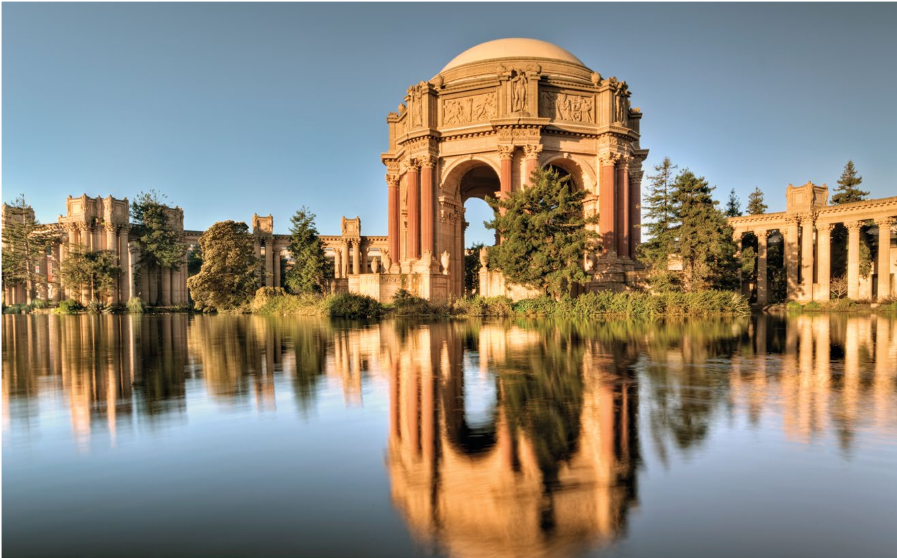
[8] The Palace of Fine Arts was designed by Bernard Maybeck and built for the 1915 Panama-Pacific Exposition in San Francisco. The pavilion was intended to be temporary and, although it had a steel structure, the exterior was finished only with stucco, an impermanent material composed of plaster and fiber. The building was not torn down after the exposition, and it eventually fell into ruin. In 1964, all but the steel structure was demolished, and the building was reconstructed with lightweight poured-in-place concrete. Photo: KevinIcole at Wikimedia Commons.
