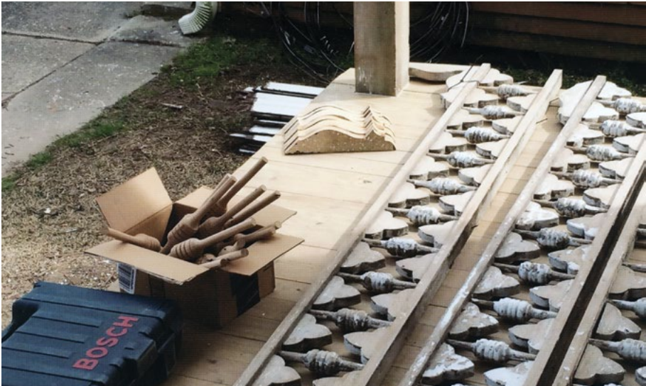
[5] New wood trim pieces were milled to match the few remaining historic features to replace those that were missing.
