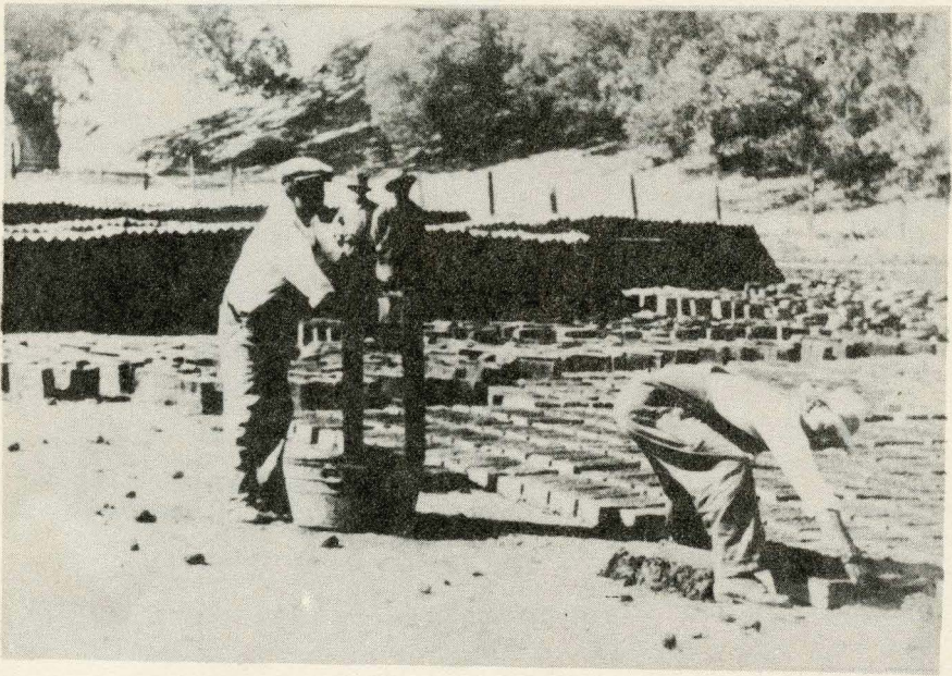
Figure 9. Method of Making Bricks. Mexicans Follow the the Time-Honored Practice, Remaking Adobe Bricks from Disintegrated Adobe Walls on the Old Fort Premises, in 1923.
