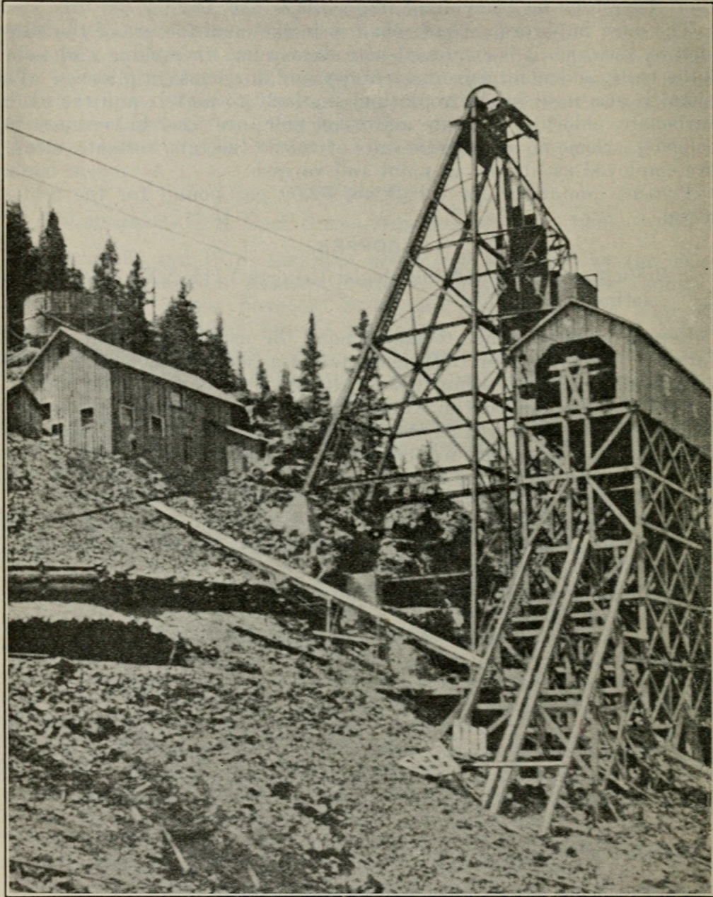
Tramway terminal and head-frame at the Superior Mine, Engels Copper Company, Plumas County.
