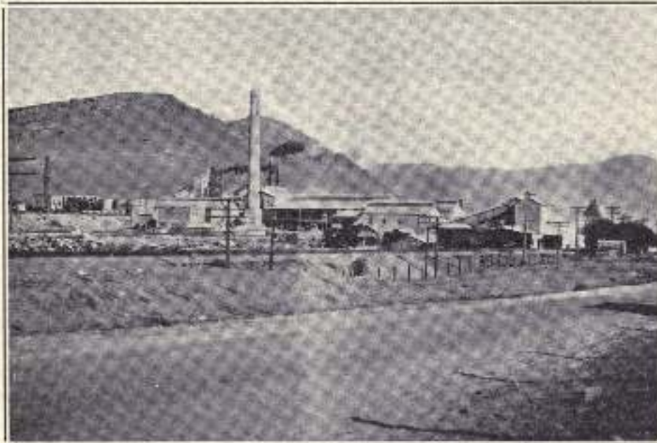
Plant of Monolith Portland Cement Company at Monolith, Kern County.
